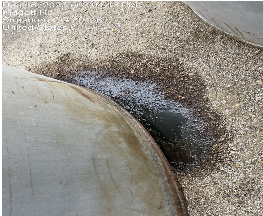
Photo 5. Photo taken of oil at the bottom of crude oil tank in tank battery. Photo taken facing north.
