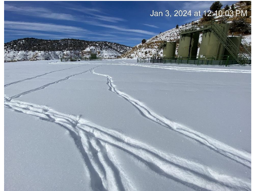
Location from Southeast corner
