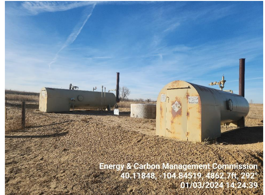
Photo 14 Horizontal Heater Treaters.
