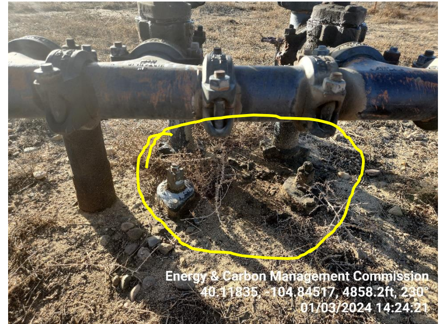
Photo 12 Stained soil by the flow line manifold.
