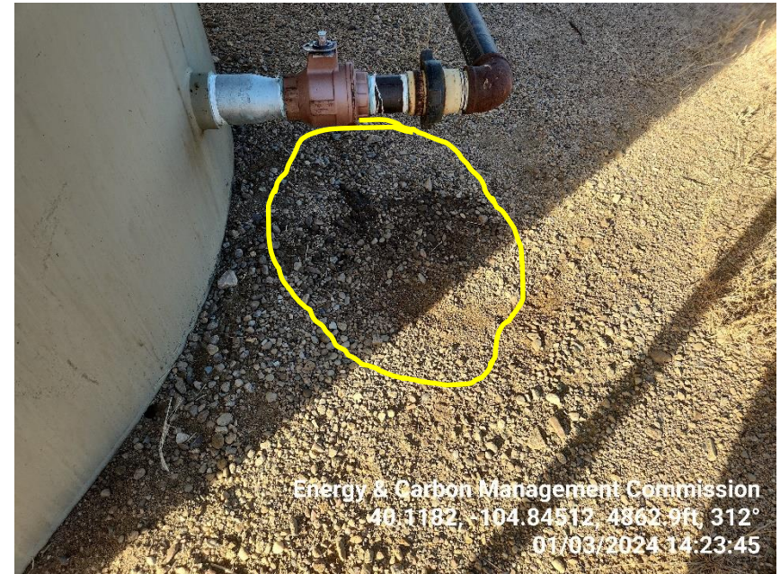
Photo 8 Stained soil by the TB load out valve
