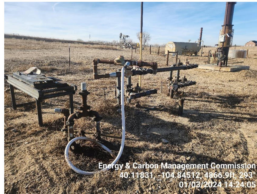
Photo 10 Flow line manifold.
