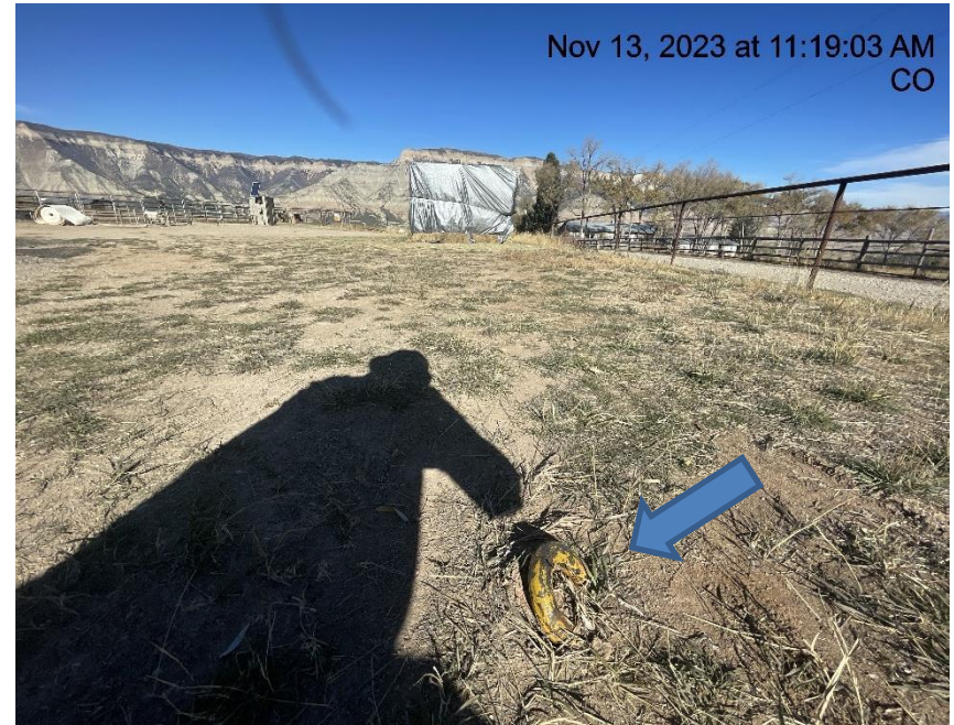
Photo # 6444 From inspection 708902222 conducted on 11/13/2023 Unmarked deadman
