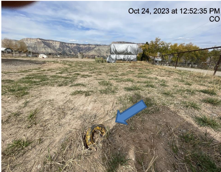
Photo # 4059 From inspection 708902036 conducted on 10/24/2023 Unmarked deadman
