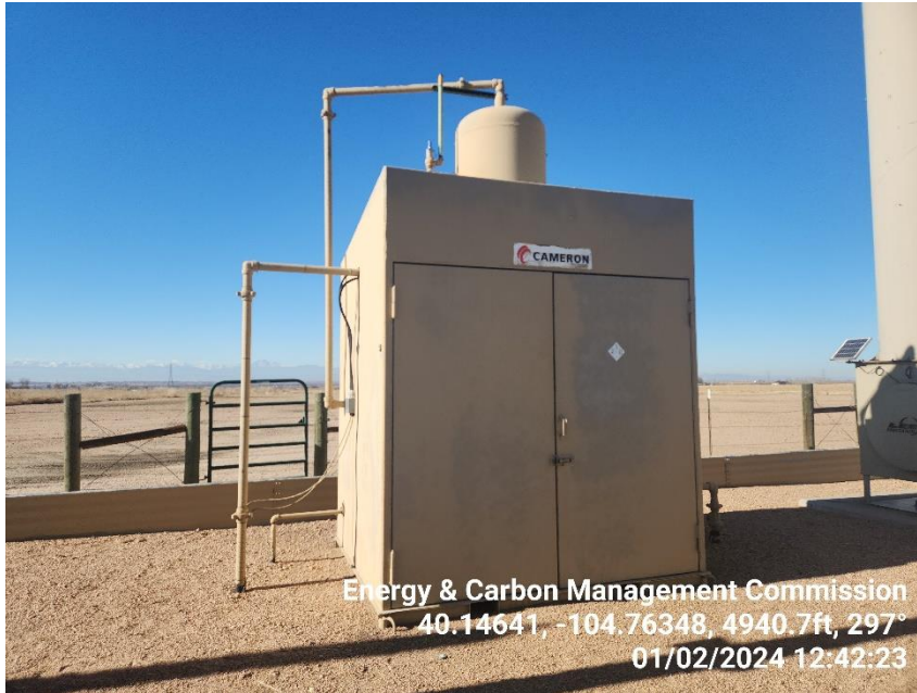
Photo 11 Vertical Separator.
