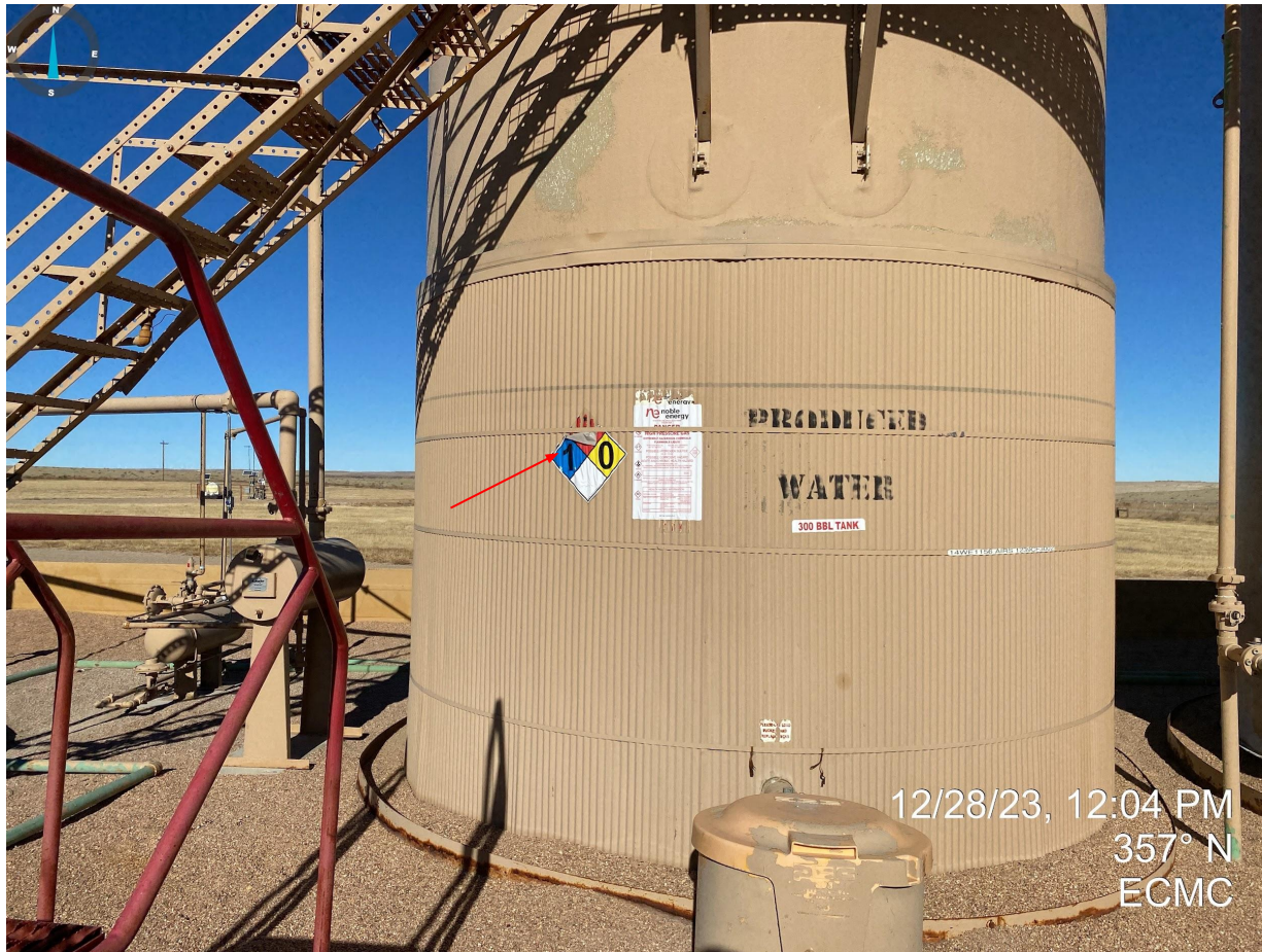
Photo 4. NFPA placard at produced water tank is not legible.
