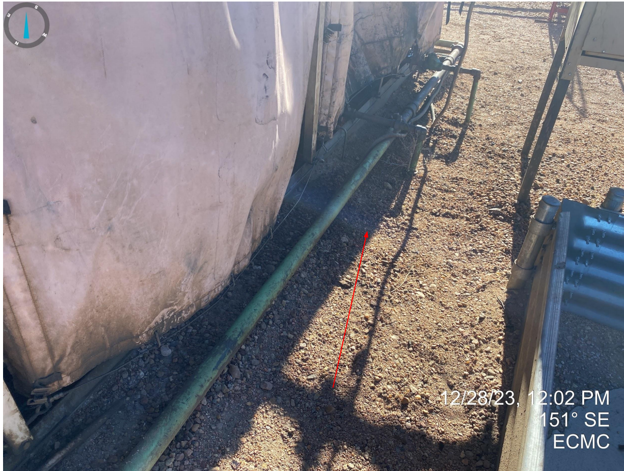
Photo 2. Stained soil observed around compressor station.
