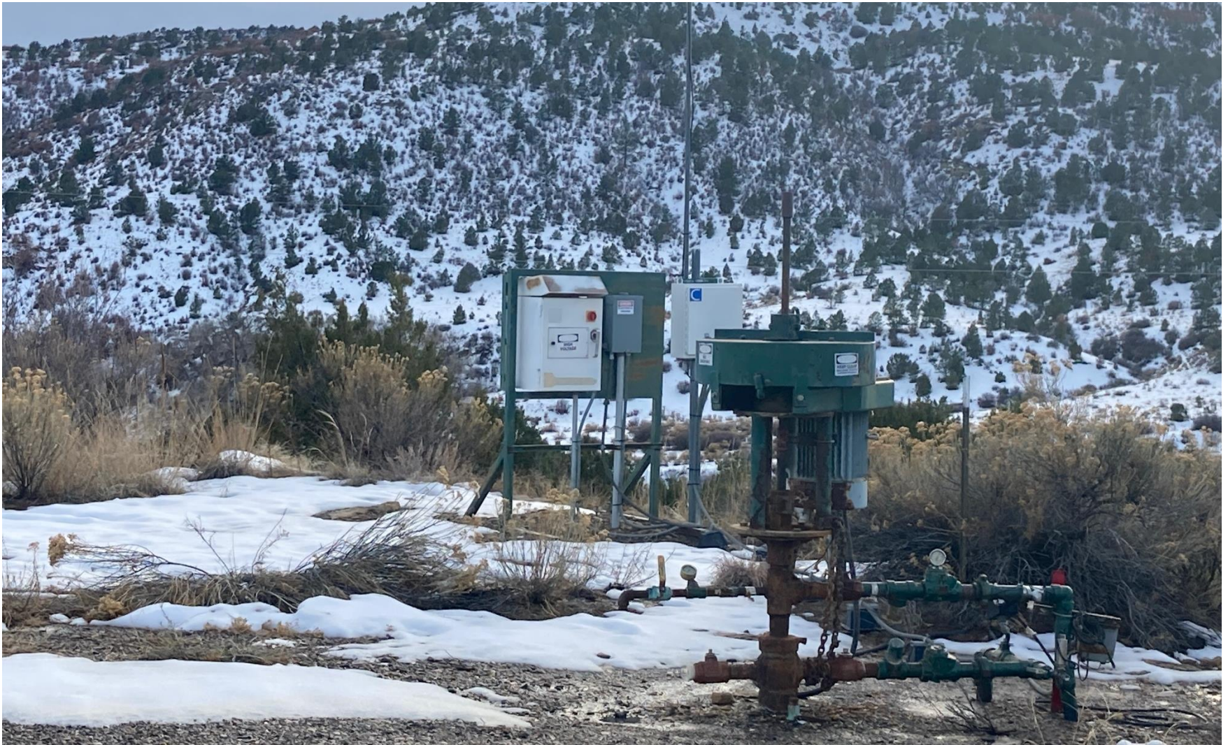
PHOTO 3: WEEDS NOT MAINTAINED AROUND WELLHEAD AND EQUIPMENT. MAINTAIN WEEDS/VEGETATION AROUND ENTIRE LOCATION PER RULE 606. CA DATE 2-2-2024.
