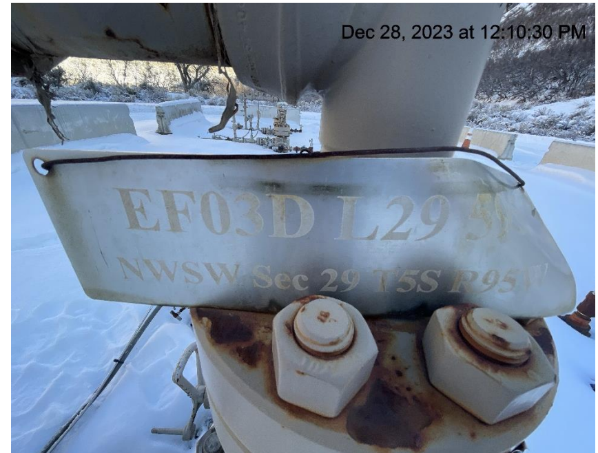
Photo # 1164 Wellhead signs lack required information
