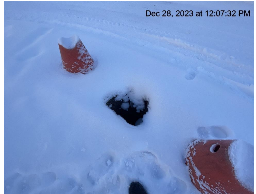
Photo # 1160 Hole near wellheads/wildlife & personnel protections insufficient (hole approximately 4-6ft deep)
