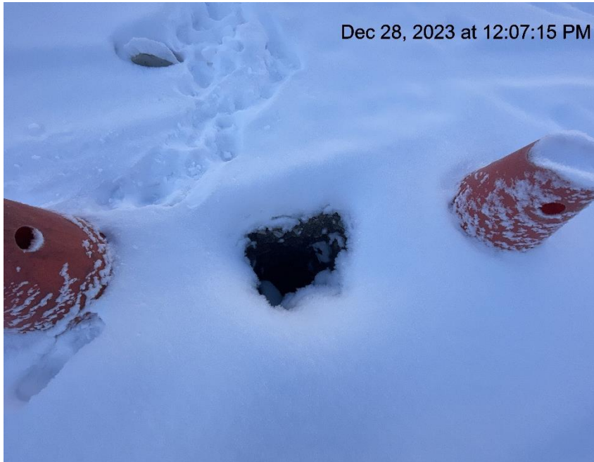
Photo # 1161 Hole near wellheads/wildlife & personnel protections insufficient (hole approximately 4-6ft deep)
