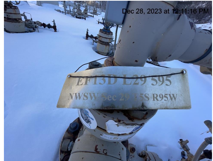
Photo # 1166 Wellhead signs lack required information
