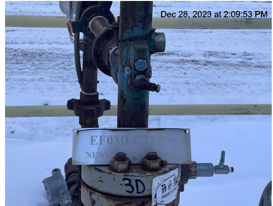
Photo # 1369 Wellhead sign lacks required info
