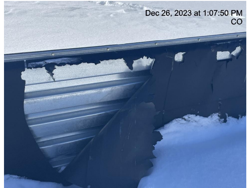
Photo # 853 Secondary containment liner needs maintenance
