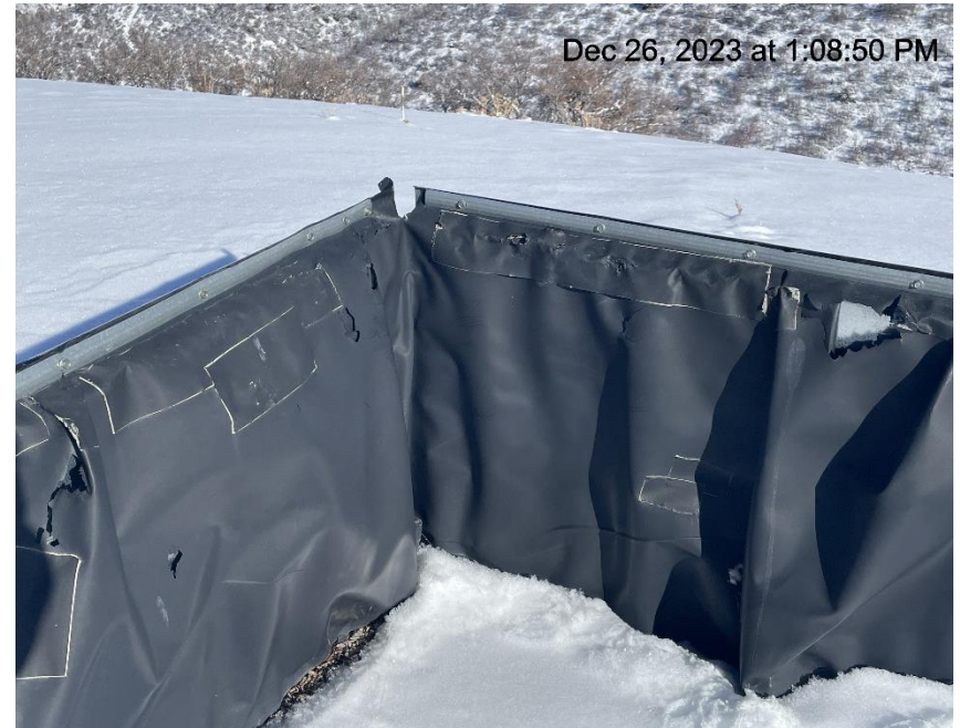
Photo # 859 Secondary containment liner needs maintenance
