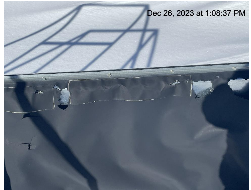
Photo # 857 Secondary containment liner needs maintenance
