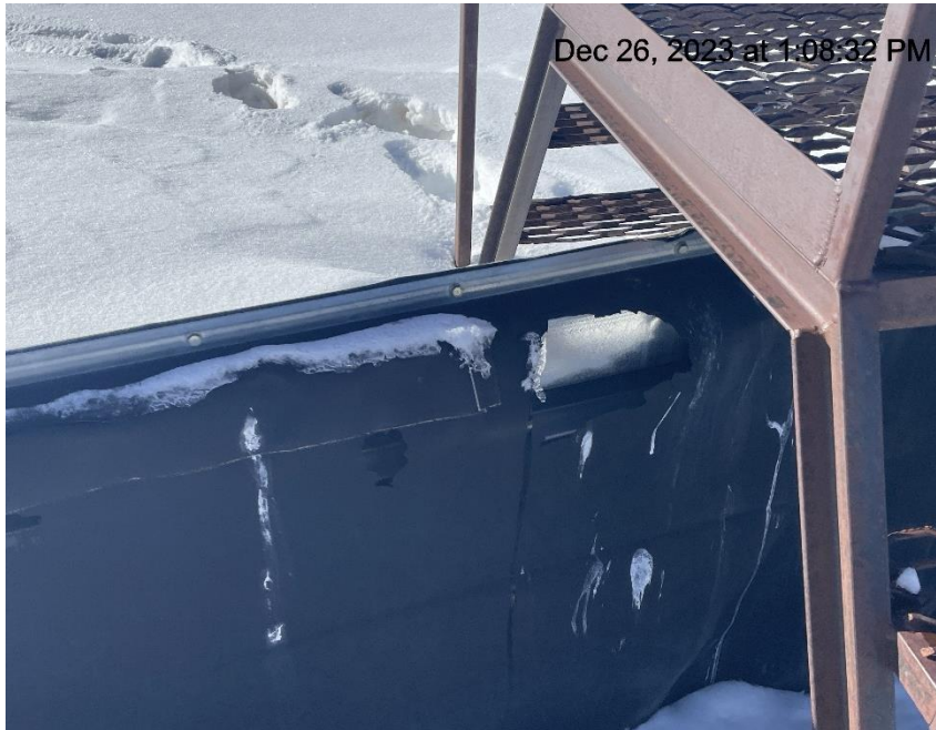
Photo # 856 Secondary containment liner needs maintenance
