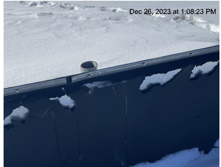
Photo # 855 Secondary containment liner needs maintenance
