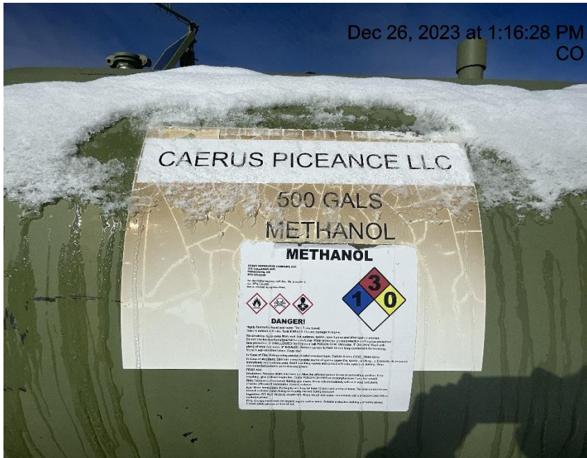
Photo # 846 Methanol tank missing required info
