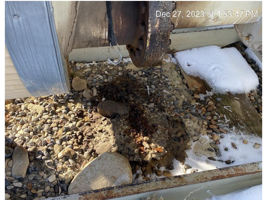
Staining below fire tube
