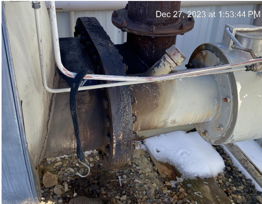
Debris. Leaking fire tube.
