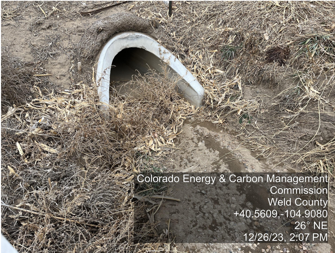
Photo 9. The photo was taken from the tank battery location facing Northeast. The photo illustrates the straw wattle protecting the culvert at the entrance needs repair.
