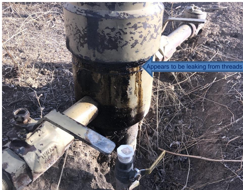
Photo # 4 Apparent leak on well head.
