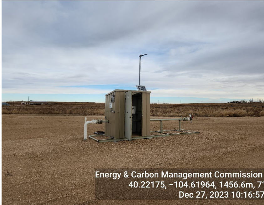
Photo 3: Unused/disconnected gas meter
