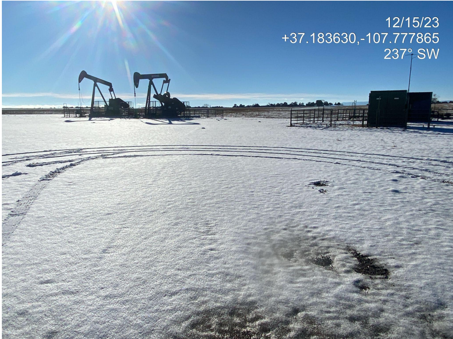
Photo 1. View of the well disturbance from the entrance facing center.
