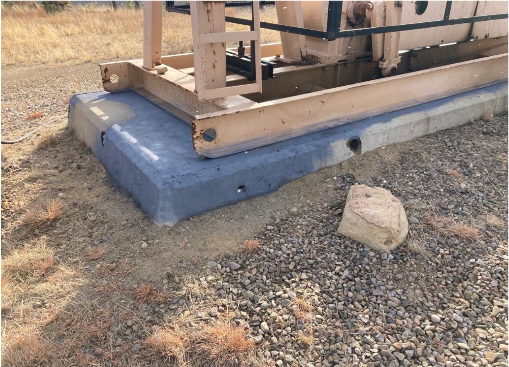
PHOTO 2: THE STAINED CONCRETE RISER HAS BEEN PAINTED THE SURROUNDING SOIL STAINS REMOVED. MECHANICAL MAINTENANCE HAS BEEN PERFORMED ON ALL EQUIPMENT.
