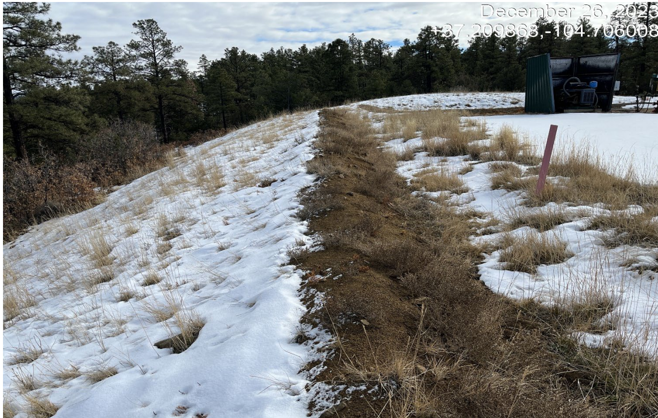
Photo 2. Facing southeast along the fill slope.
