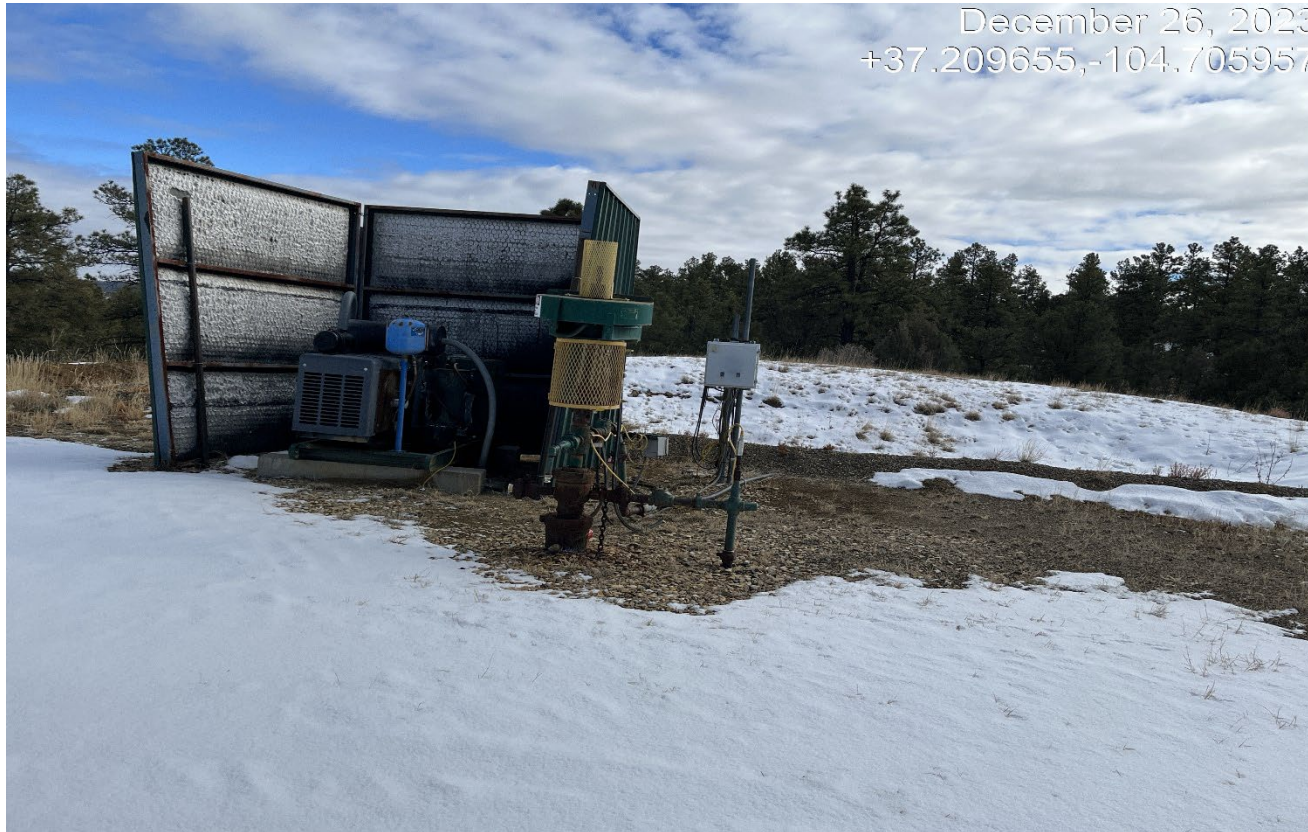
Photo 3. Facing toward the wellhead..
