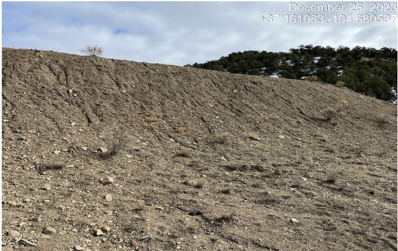
Photo 8. The embankment of the pre-existing pit is not stabilized and should be vegetated for long-term stabilization.
