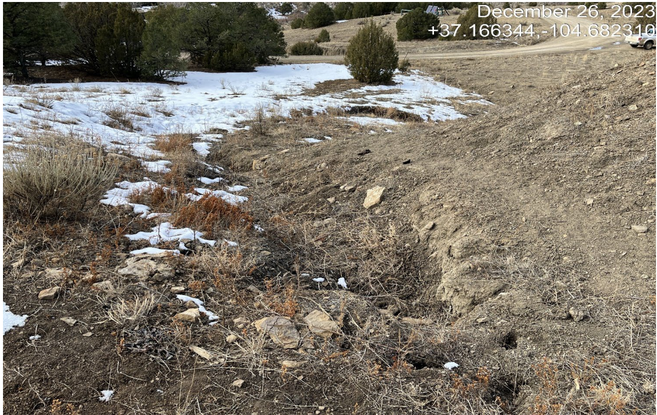
Photo 7. There is erosion along this area where water is discharged in storm events. This area should be armored and stabilized.
