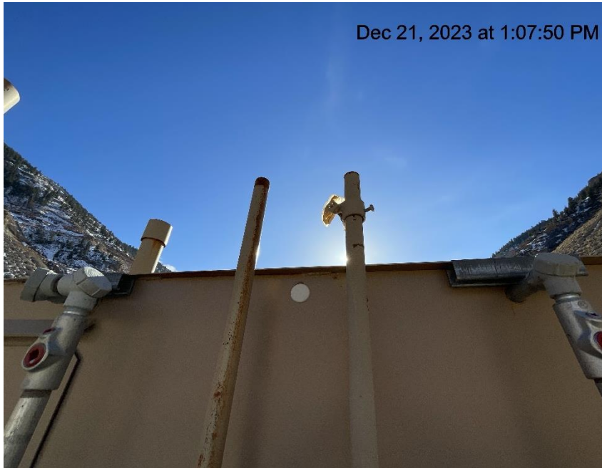
Photo # 697 PRV & Rupture disc vent lines lack caps
