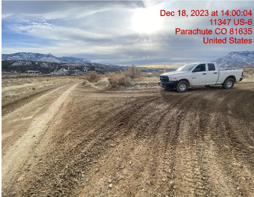
Insufficient Vehicle Tracking BMPs at Location Entrance/Exit – Photo #08300
