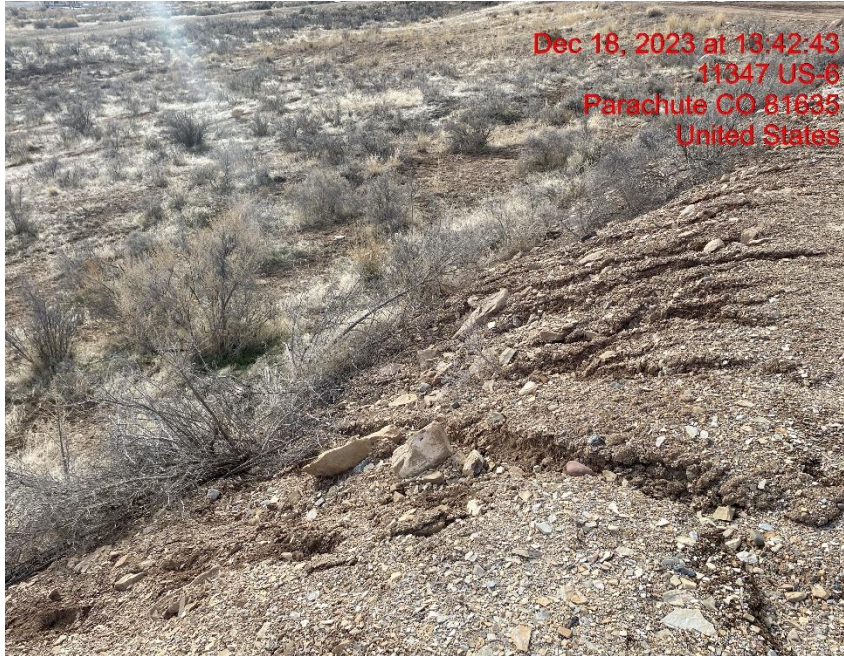
Rill Erosion Transporting Sediment Off Location – Photo #08280
