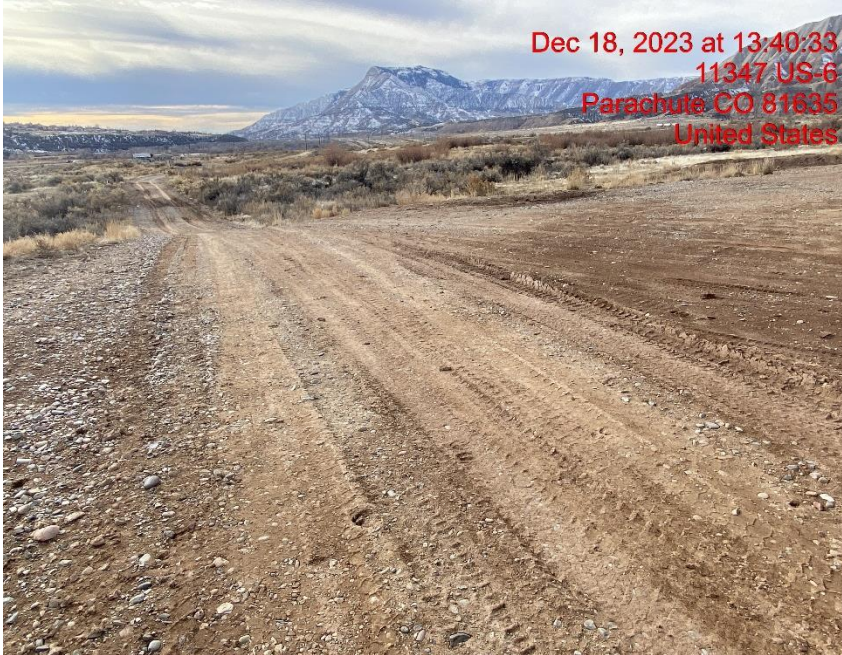
Insufficient Vehicle Tracking BMPs at Location Entrance/Exit – Photo #08275
