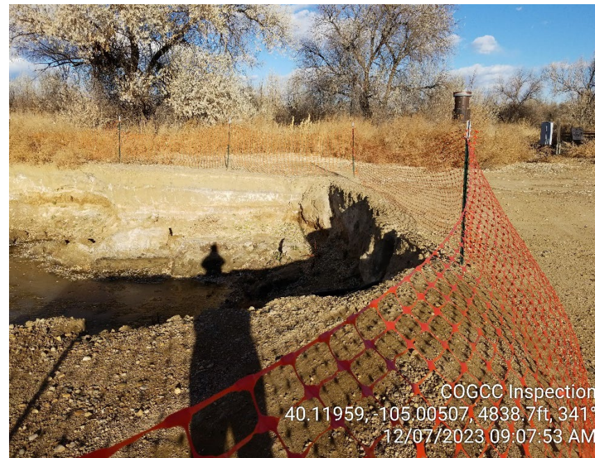
Photo 14 - Open excavation with salt crust.
