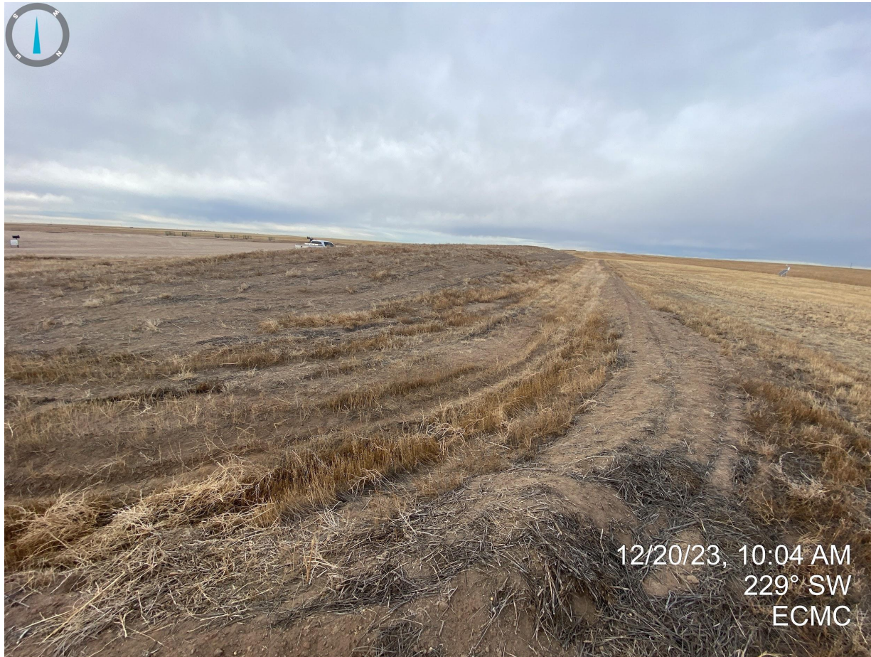
Photo 2. Taken from the northeast corner of the location. Photo illustrates that a perimeter stormwater control (ditch and berm) has been constructed around the entire perimeter of the disturbance area. Also pictured, the eastern side of the topsoil stockpile.
