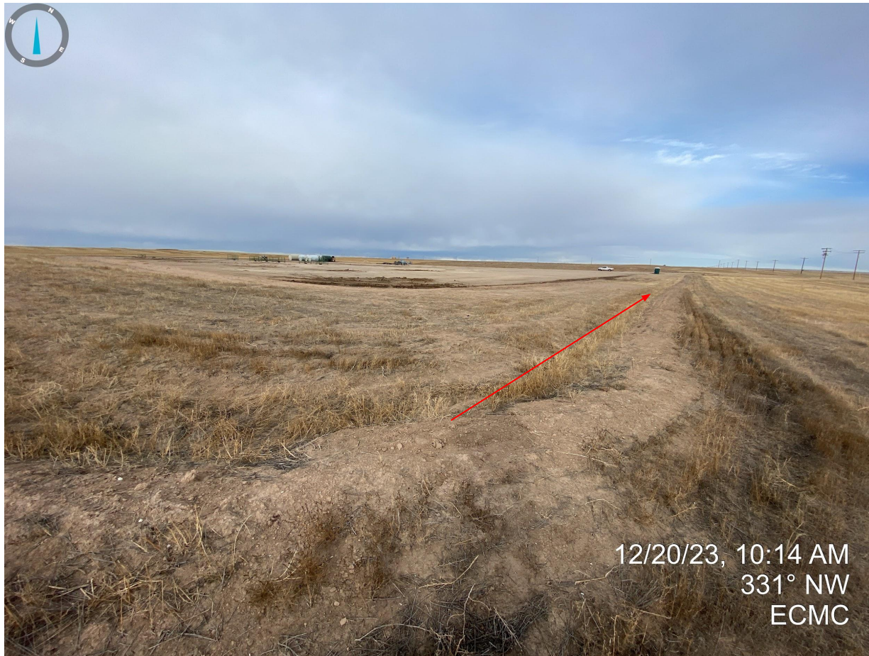
Photo 11. Taken from the southeast corner of the disturbance area. Photo illustrates that the temporary stormwater ditch and berm has been installed throughout the entire perimeter of the location.
