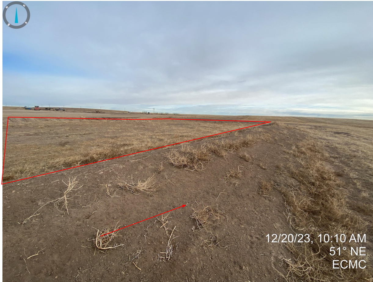
Photo 9. Red outlined area represents the stormwater detention area. Portions of the earthen berms require additional stabilization techniques to prevent wind and water erosion as they are comprised of bare/exposed soils.
