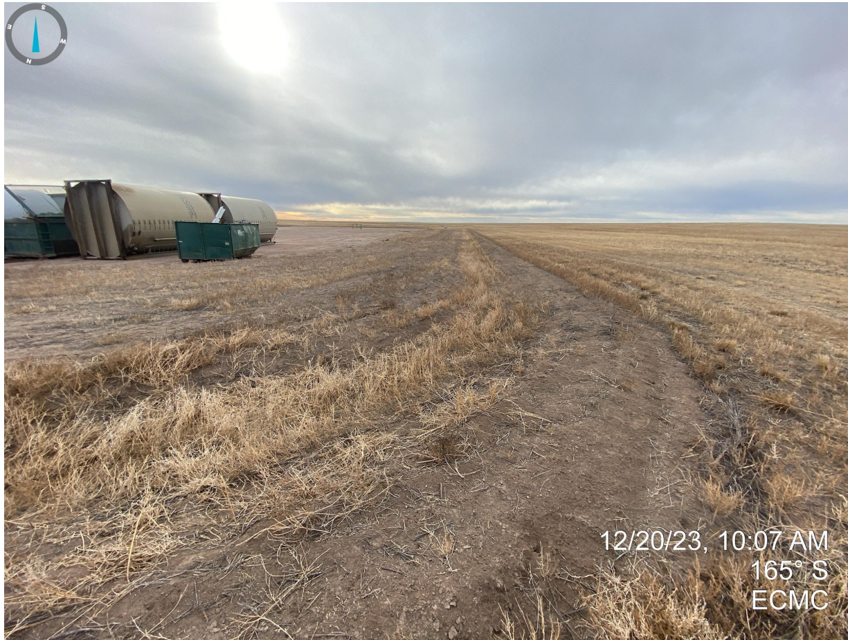
Photo 7. Taken from the northwest corner of the disturbance area. A temporary stormwater control/BMP (ditch and berm) has been constructed around the entire perimeter of the location.
