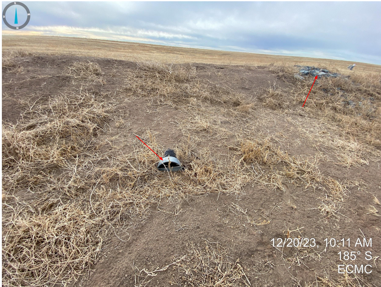
Photo 10. Taken within the stormwater detention area. Photo illustrates the outflow culvert and rip rap overflow. See also comments in previous photo.
