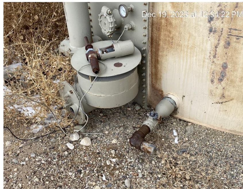
Debris. Igniter hole open to wildlife
