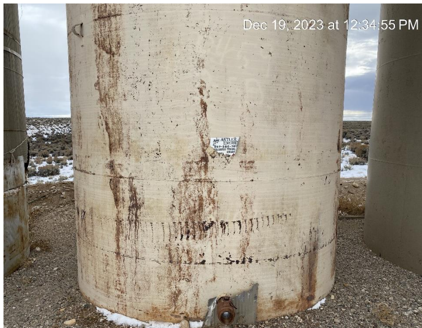
Peeled and illegible label. Open end tank valve
