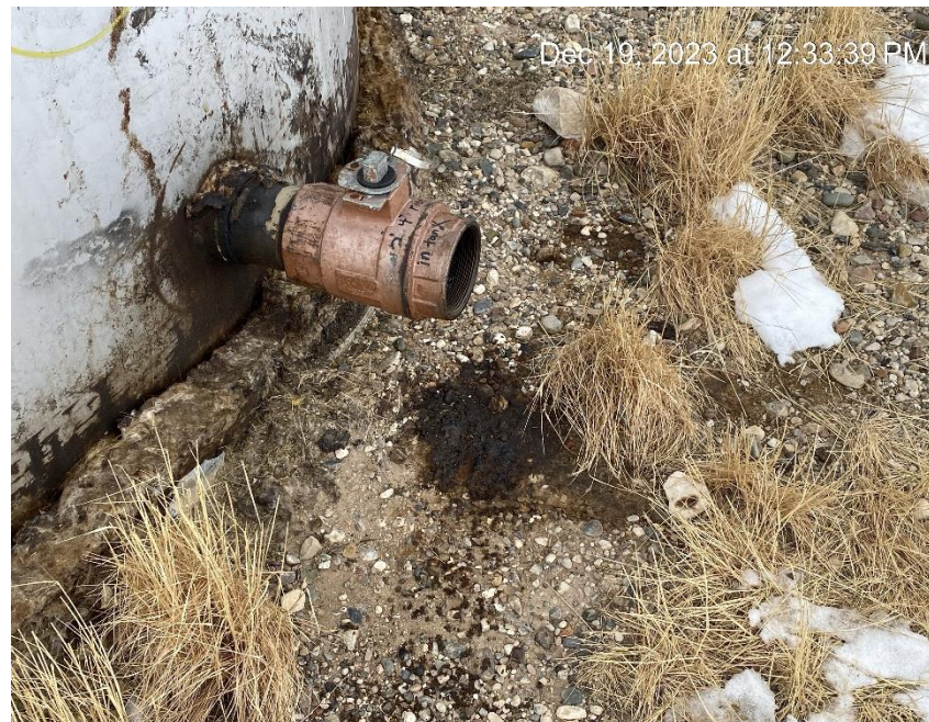
Open end tank valve. Spill
