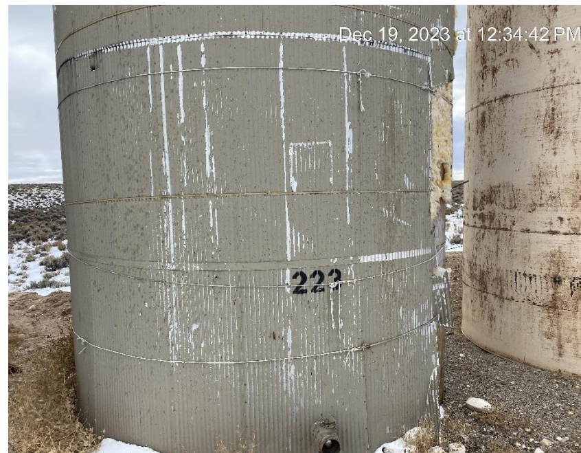
Unlabeled tank. Open end tank valve.
