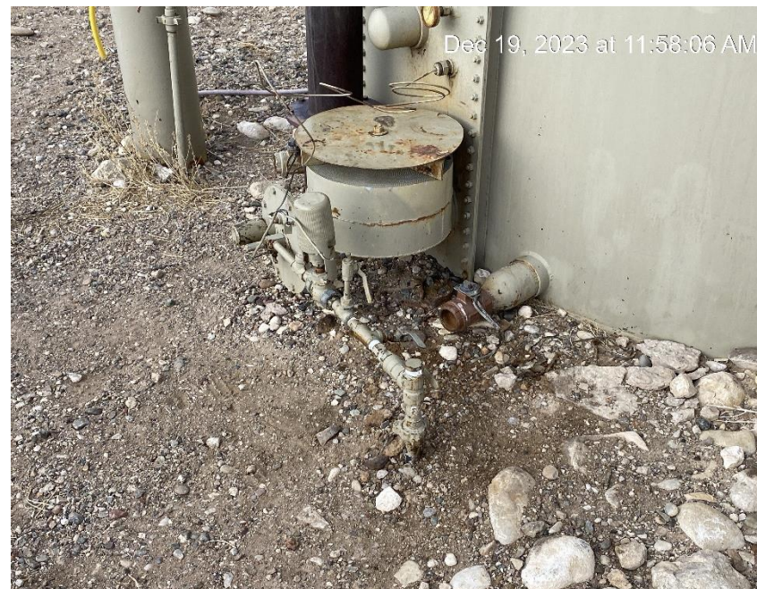
Open end tank valve still lacking plug
