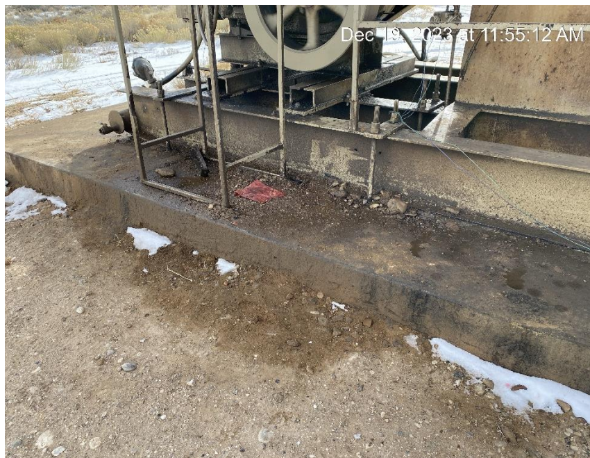
Unit still leaking oil on equipment and into soil
