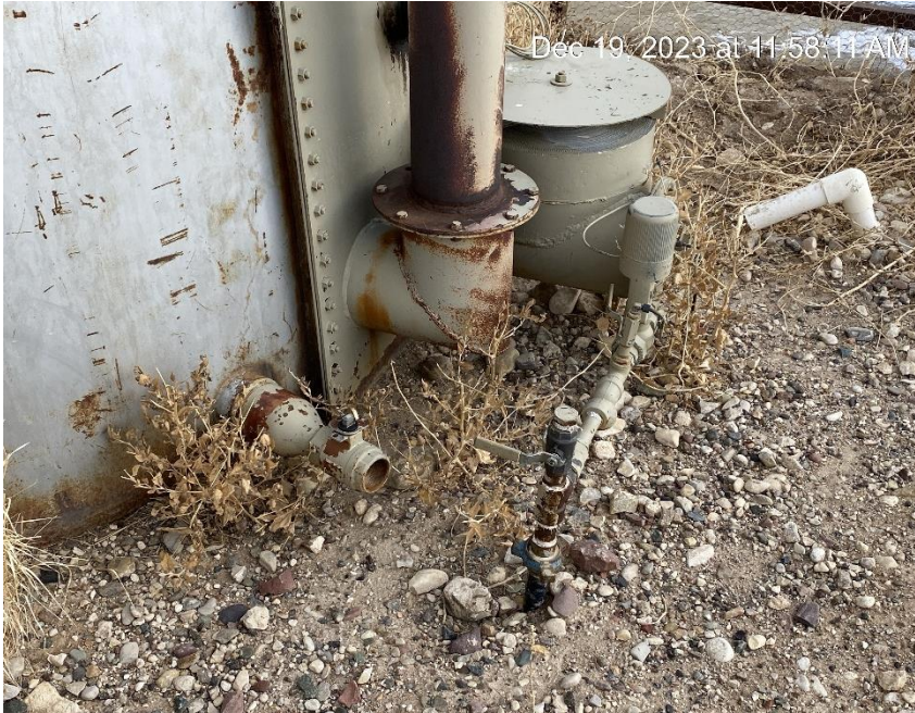
Open end tank valve still lacking plug
