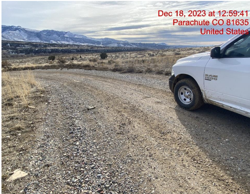
Insufficient Vehicle Tracking BMPs at Location Entrance/Exit – Photo #08245
