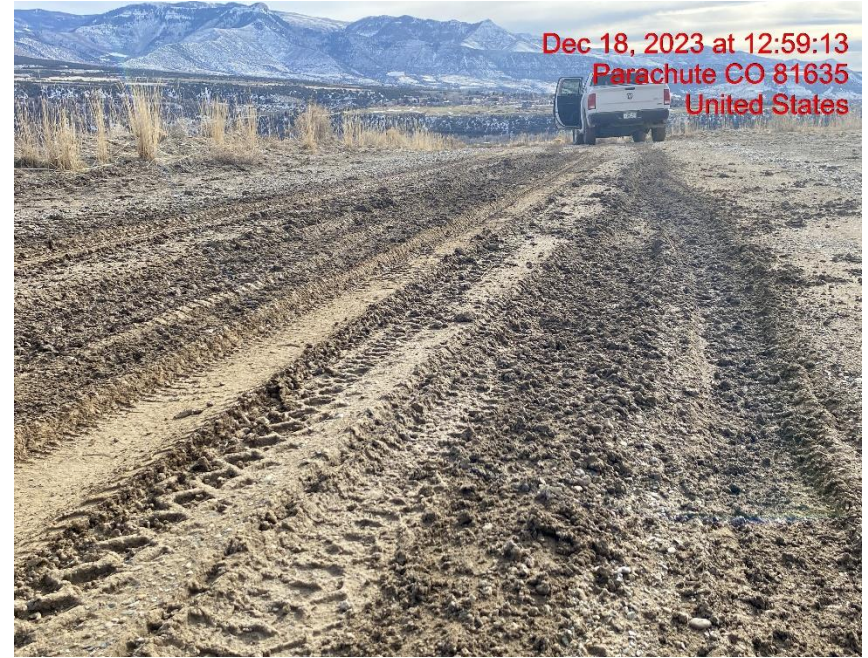
Lack of Stabilization – Photo #08244
