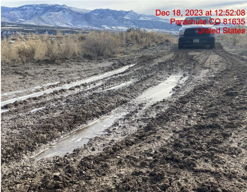
Lack of Stabilization – Photo #08237
