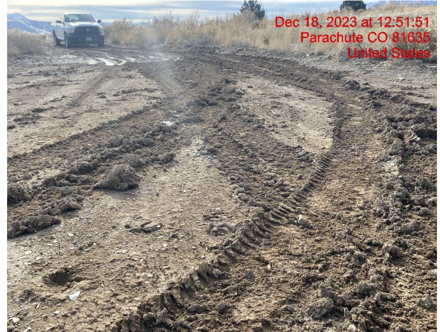
Lack of Stabilization – Photo #08236
