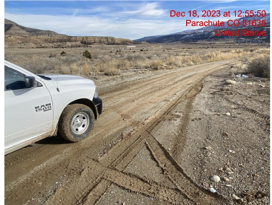
Insufficient Vehicle Tracking BMPs at Location Entrance/Exit – Photo #08240
