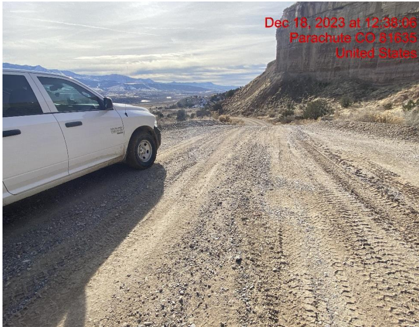
Insufficient Vehicle Tracking BMPs at Location Entrance/Exit – Photo #08224
