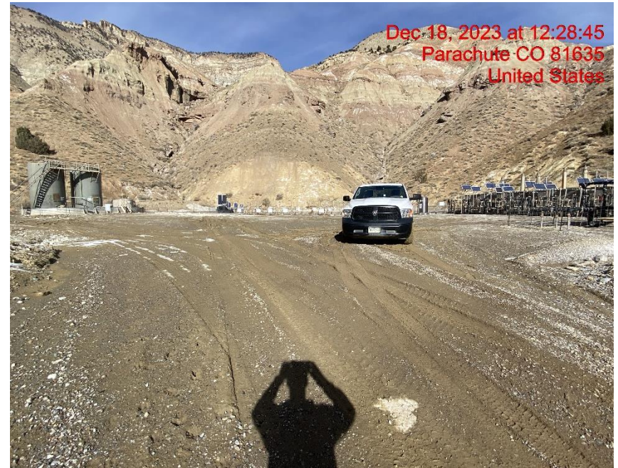
Insufficient Vehicle Tracking BMPs at Location Entrance/Exit – Photo #08213
