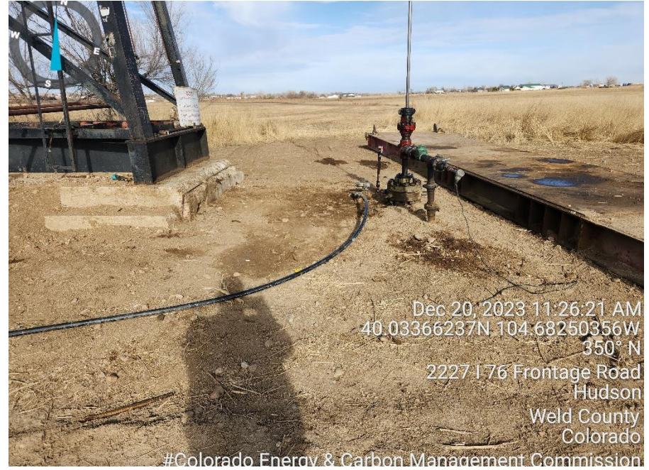
Photo 6 Stained soil around well head
