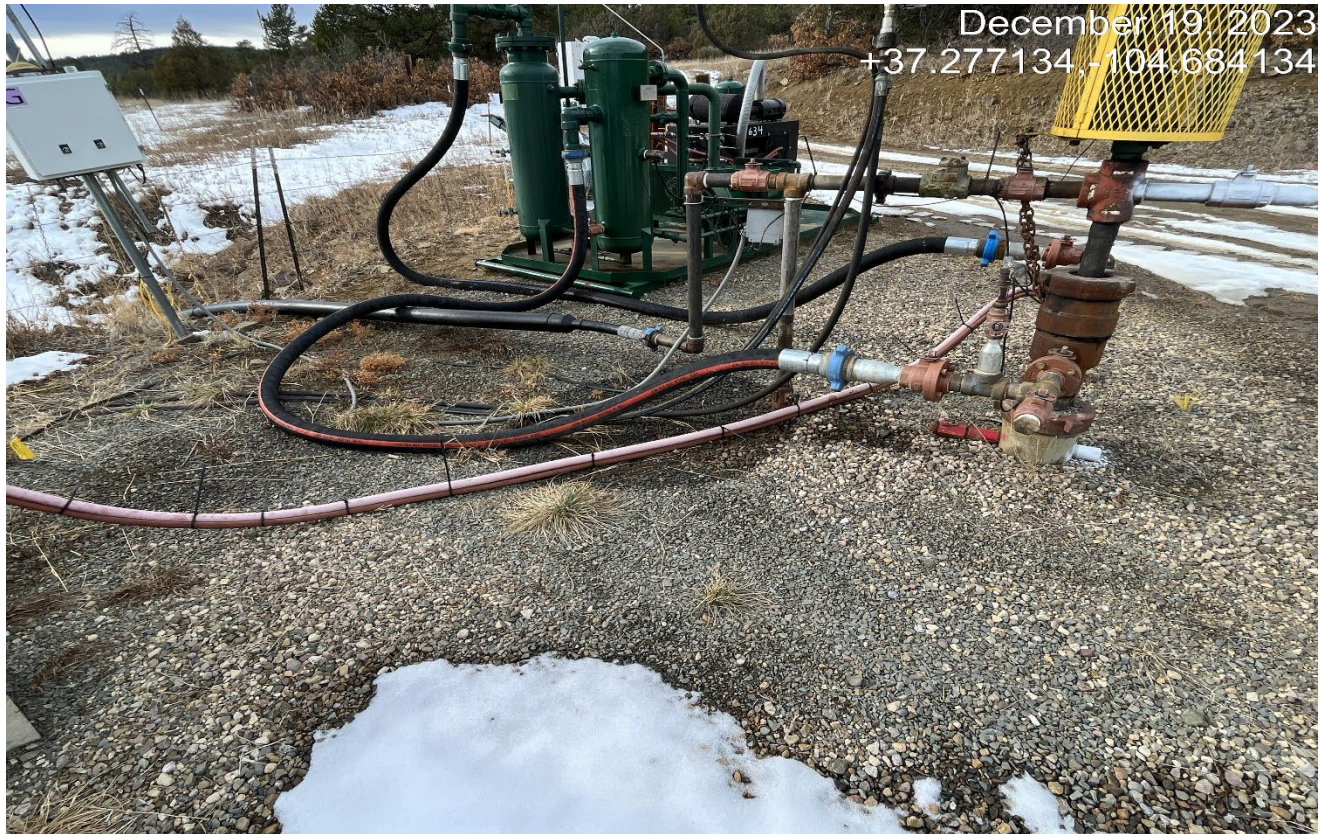
Photo 4. There is stained soils by the wellhead that will need to be cleaned up.
