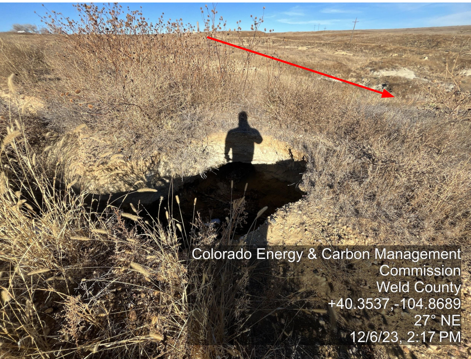
Photo 5. The photo was taken along the access road facing Northeast. The photo illustrates a large gully erosional feature that has blown out the road and run into the drainage below.
