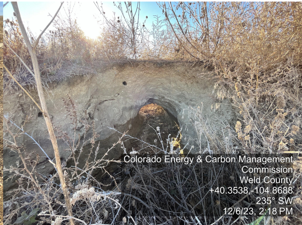
Photo 6. The photo was taken below the access road facing Southwest. The photo illustrates the bottom side of the road blow out described in photo 5.
