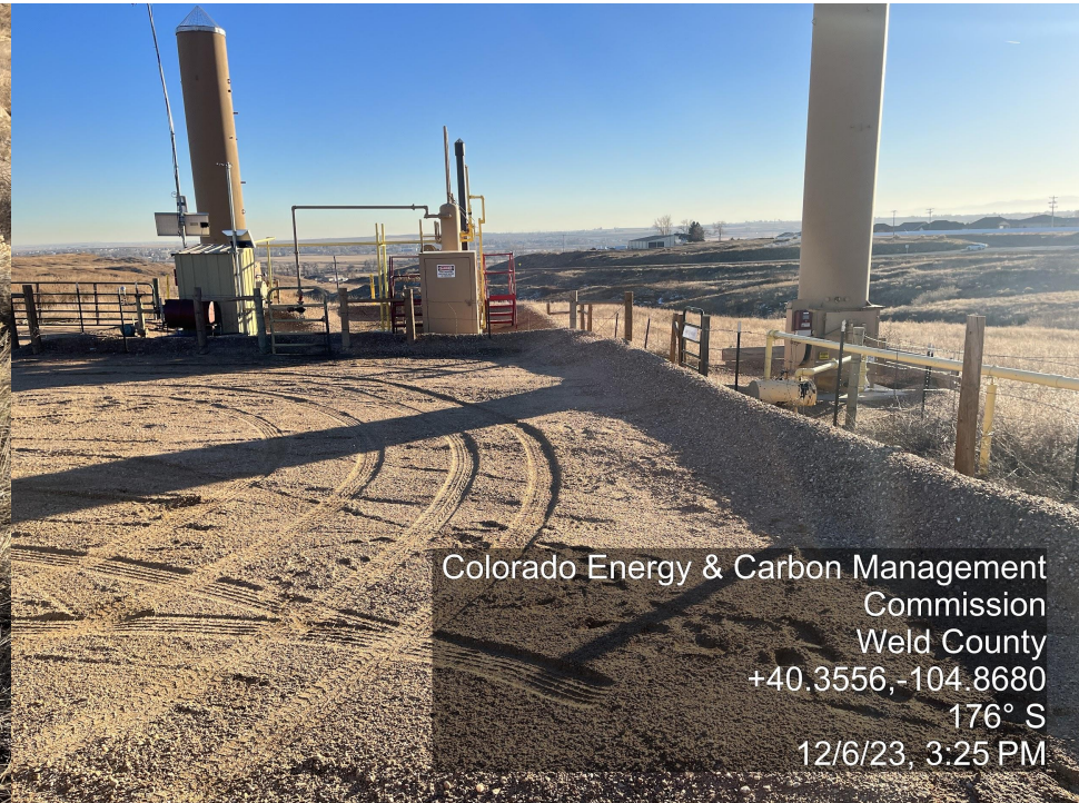
Photo 10. The photo was taken at the tank battery location facing South. The photo illustrates proper fencing as well as a gravel berm surrounding the location.
