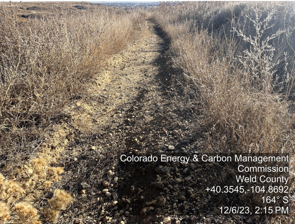
Photo 3. The photo was taken along the access road facing South. The photo illustrates pervasive erosion that ran along the majority of the access road.
