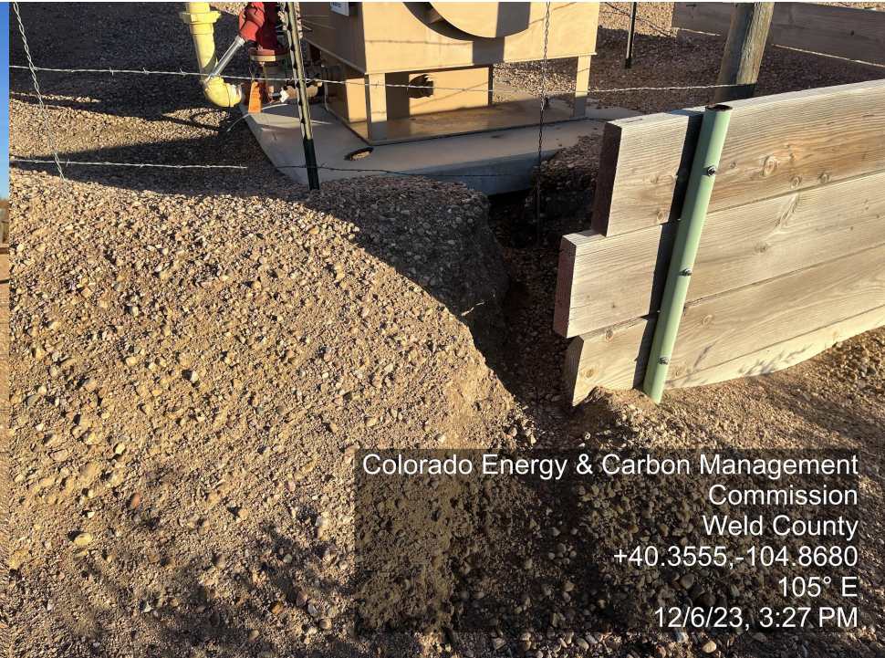
Photo 12. The photo was taken at the tank battery location facing East. The photo illustrates erosion occurring under the concrete pad of some oil and gas equipment.
