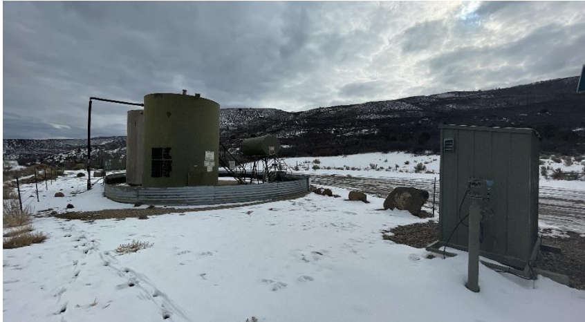
North West corner of location.
