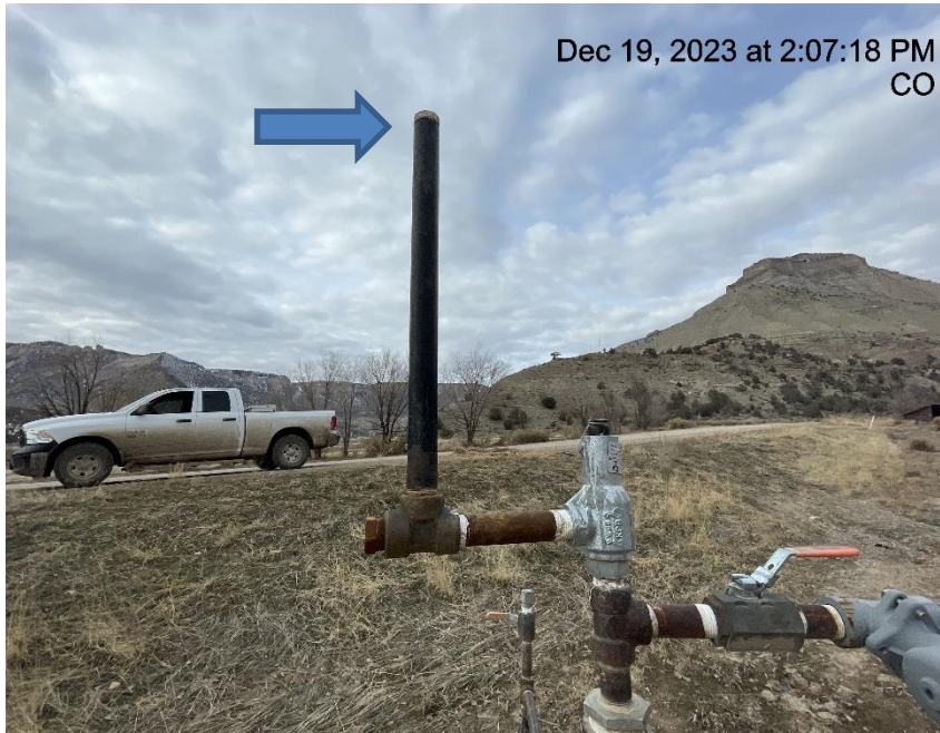
Photo # 384 PRV vent line lacks cap
