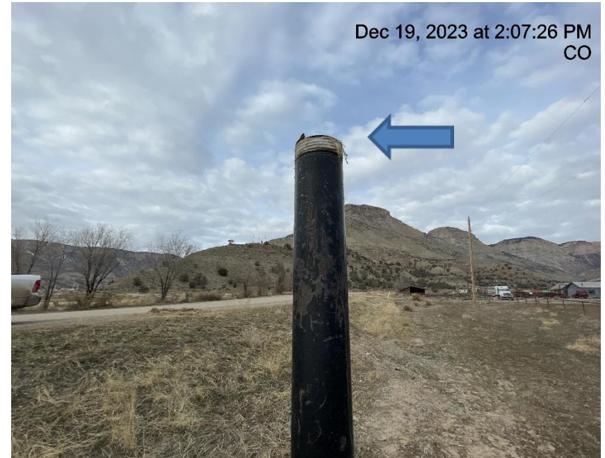
Photo # 385 PRV vent line lacks cap
