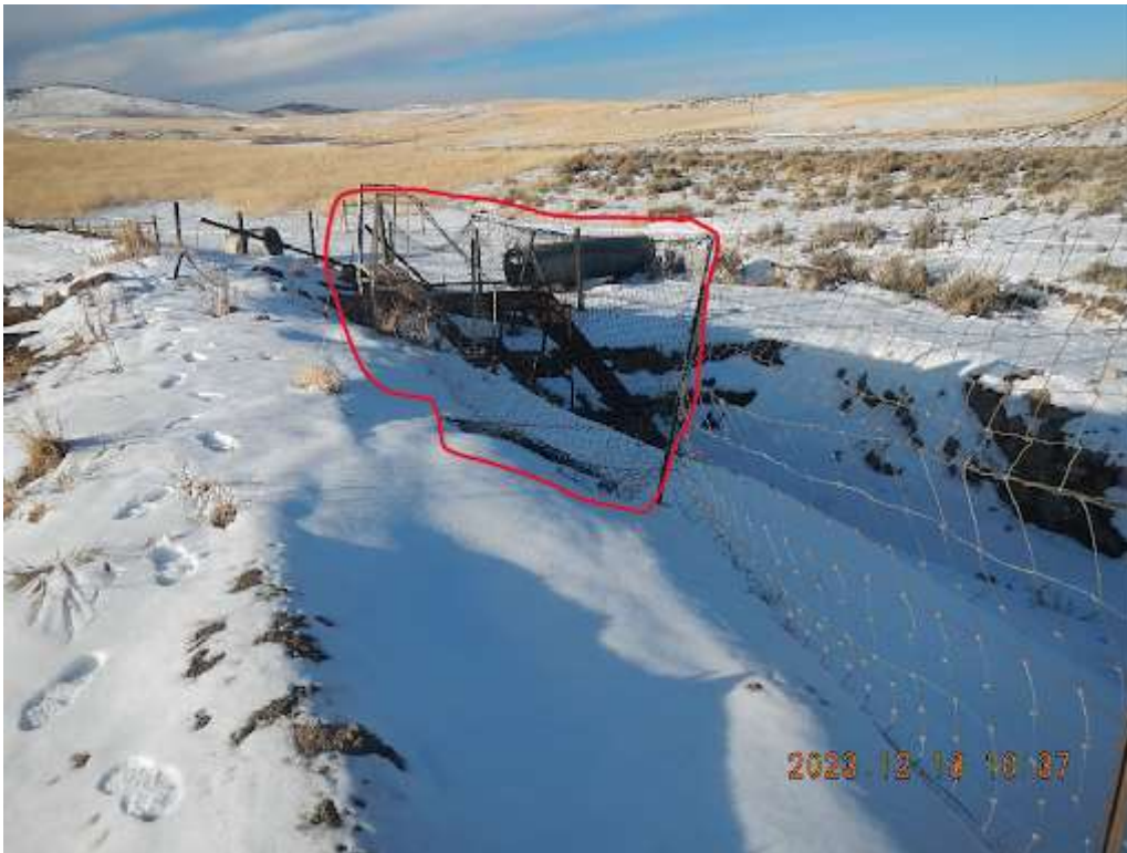
Oil accumulation in Pit Facility ID: 116587. NOTE: No bird netting present.
