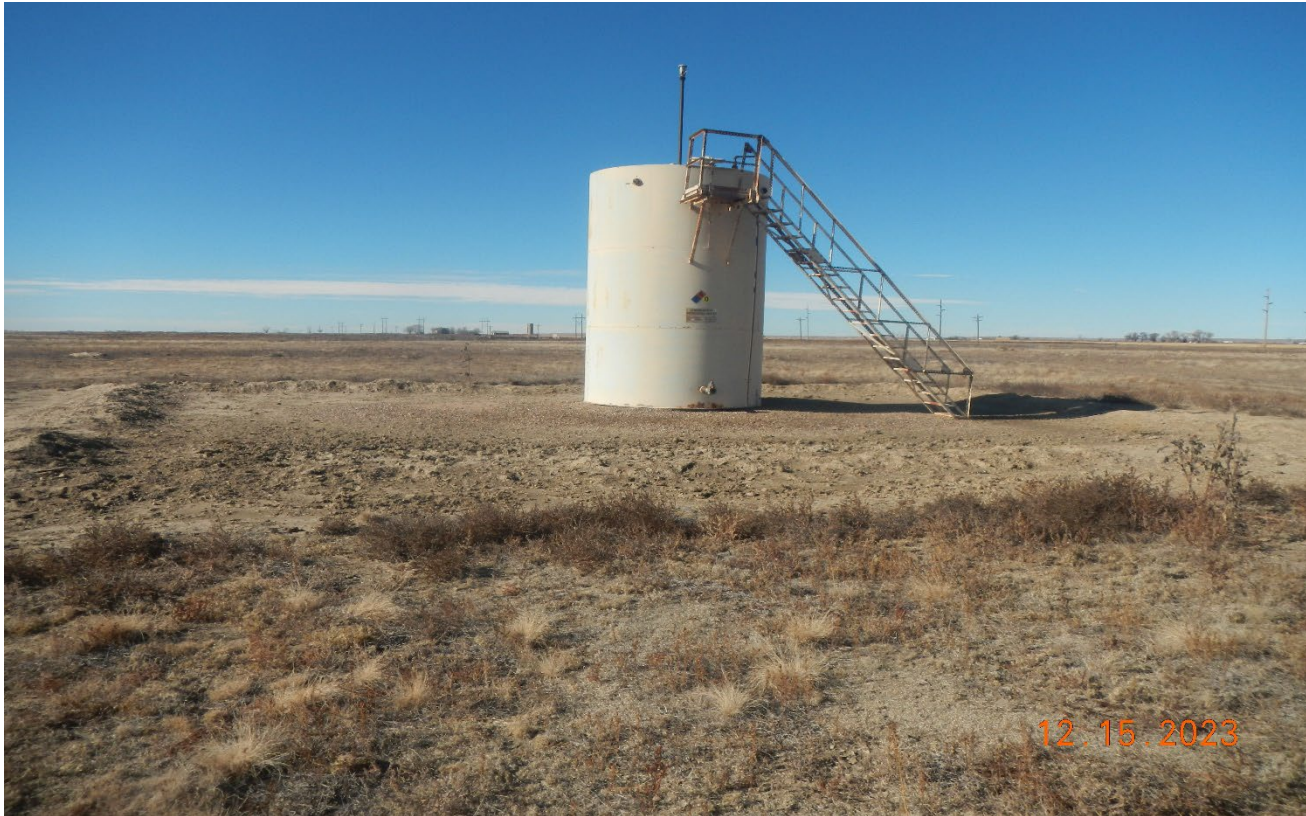
Photo 2. Facing toward the tank battery. There is insufficient secondary containment to contain a spill.
