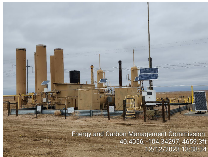
Photo 8 – Separators and ECDs
