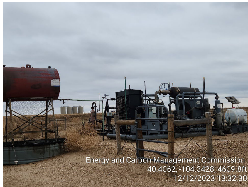
Photo 2 – Compressor – Day Tank Netting has been repaired
