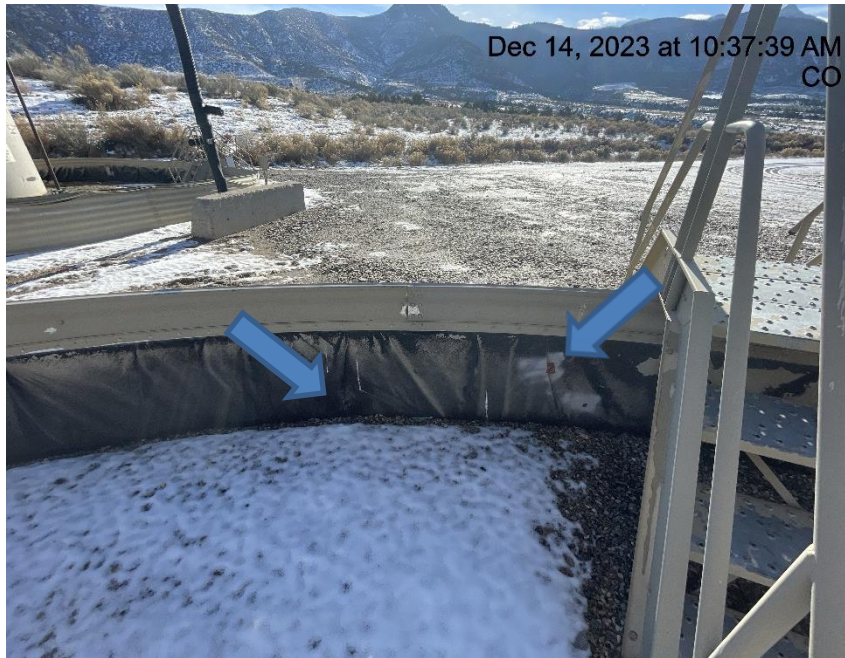
Photo # 9707 Holes in liner/liner needs maintenance (single tank containment)
