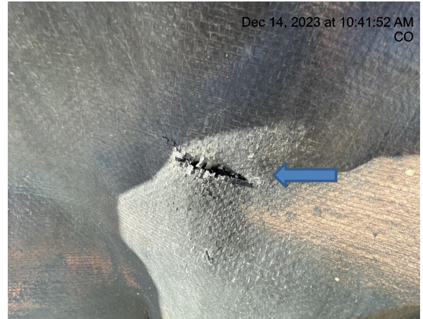
Photo # 9706 Hole in liner/liner needs maintenance (3 tank containment)
