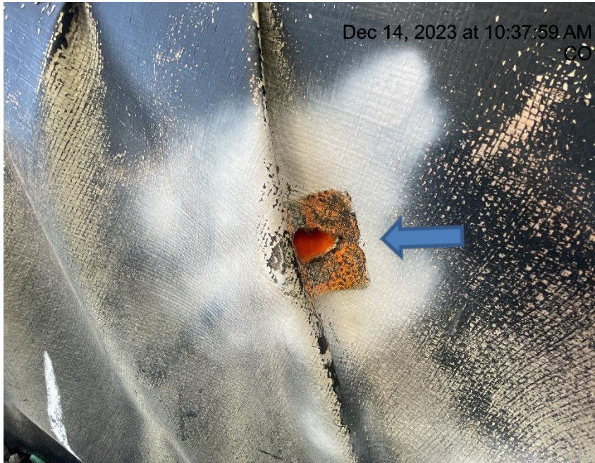
Photo # 9709 Hole in liner/liner needs maintenance (single tank containment)
