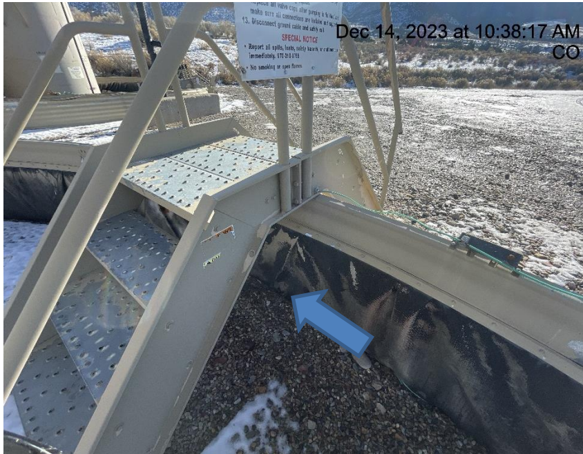
Photo # 9703 Hole in liner/liner needs maintenance (single tank containment)
