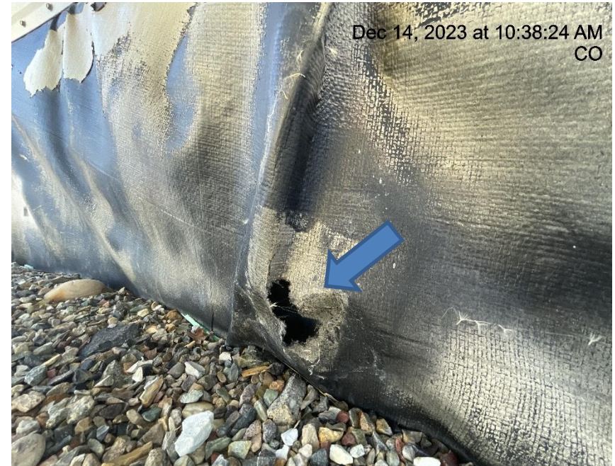
Photo # 9704 Hole in liner/liner needs maintenance (single tank containment)
