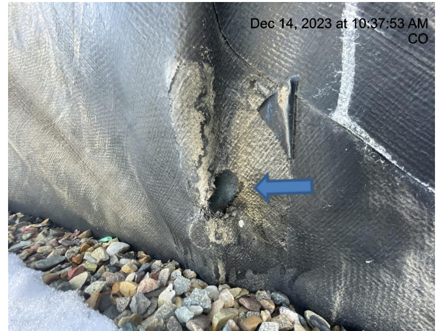
Photo # 9708 Hole in liner/liner needs maintenance (single tank containment)
