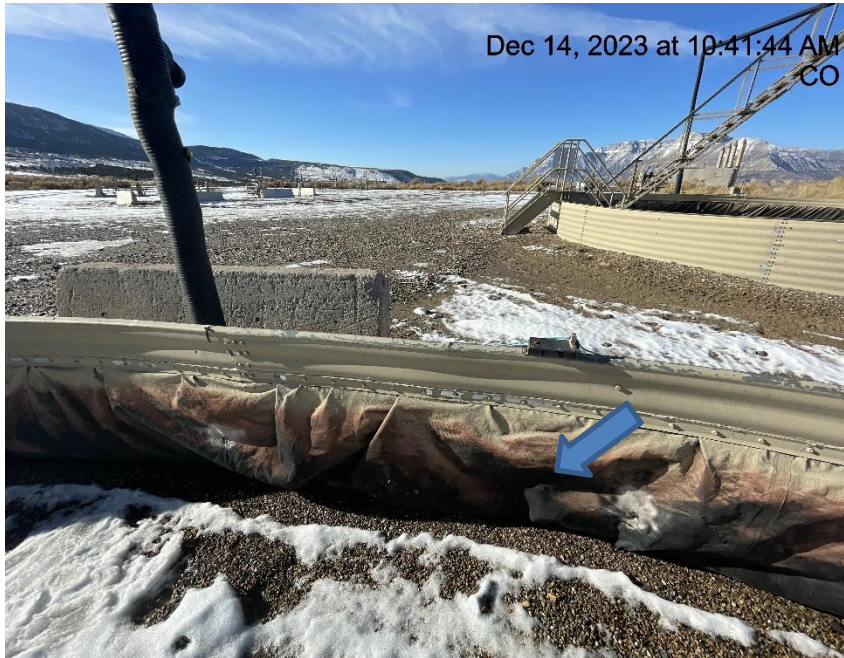
Photo # 9705 Hole in liner/liner needs maintenance (3 tank containment)
