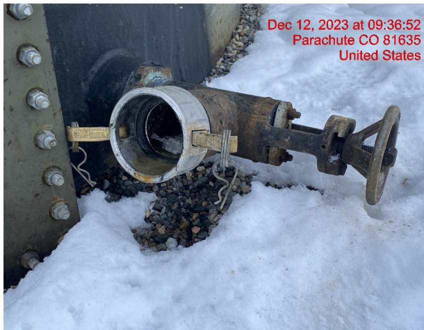
Leaking and Uncapped Load Line – Photo #08147
