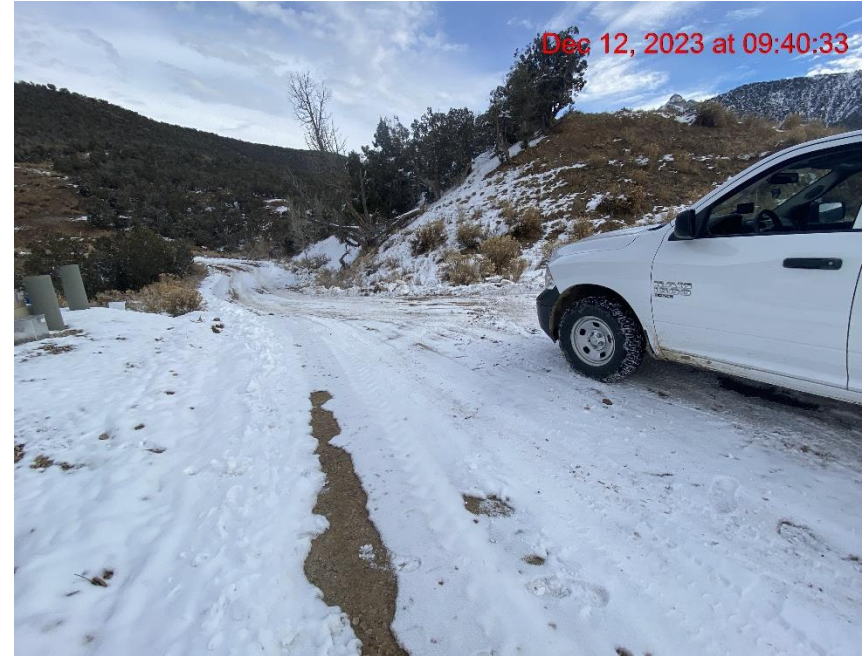
Insufficient Vehicle Tracking BMPs at Location Entrance/Exit – Photo #08154
