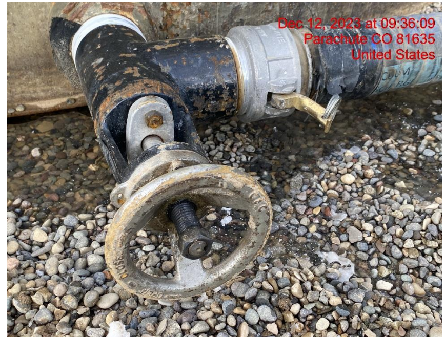
Leaking Load Line Connection – Photo #08146
