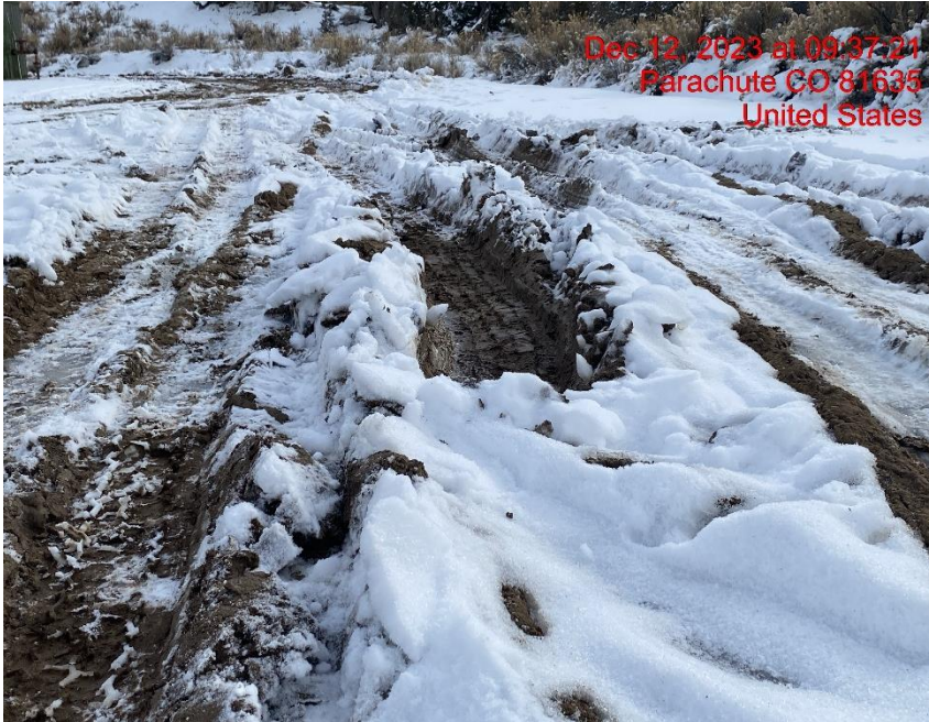
Lack of Stabilization – Photo #08148
