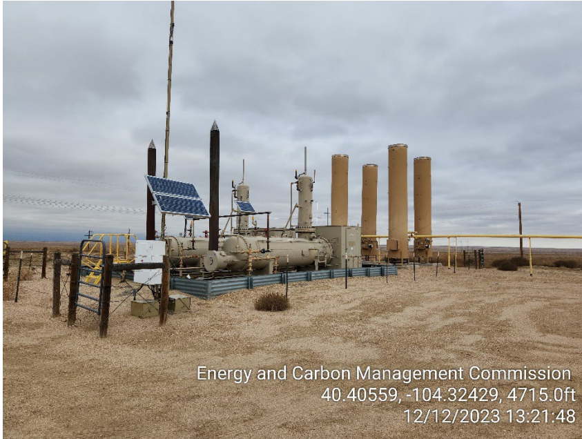
Photo 1 – Separators and ECDs
