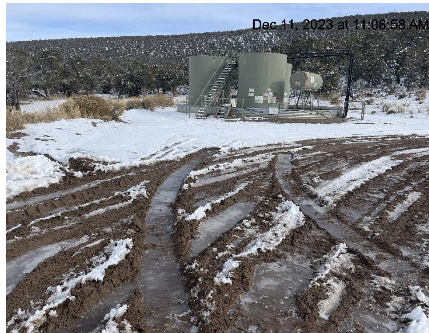
Photo # 9196 Lack of stabilization/compaction/insufficient BMP's
