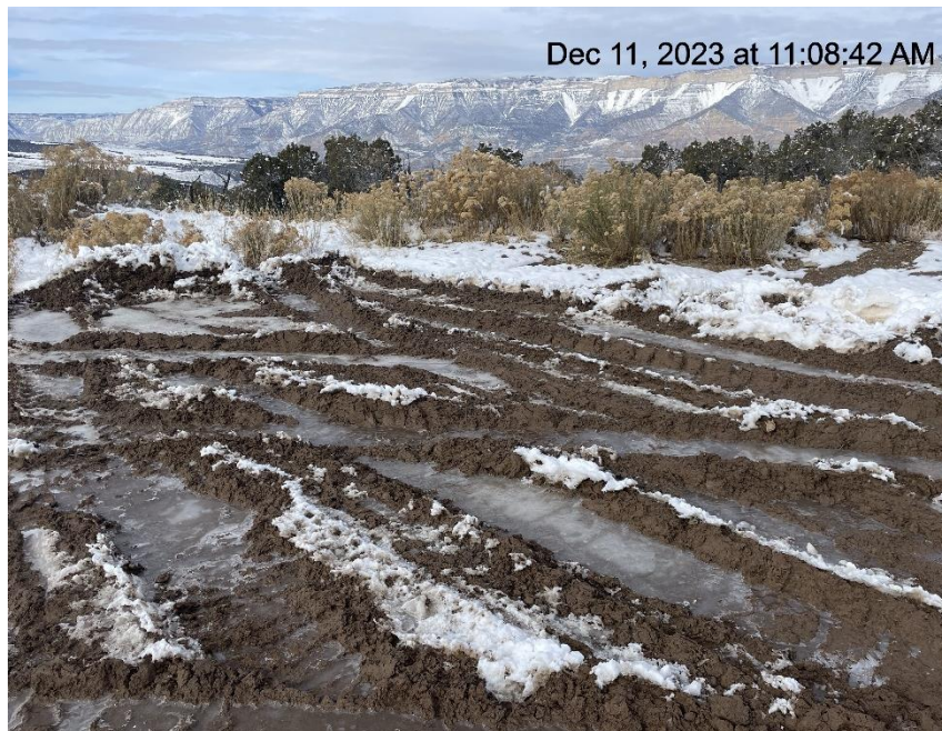
Photo # 9195 Lack of stabilization/compaction/insufficient BMP's
