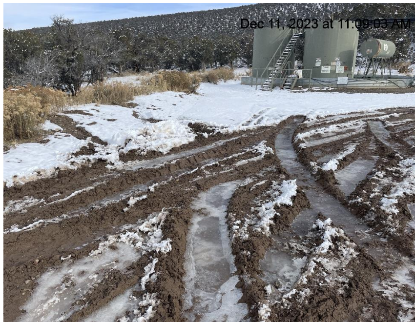
Photo # 9197 Lack of stabilization/compaction/insufficient BMP's
