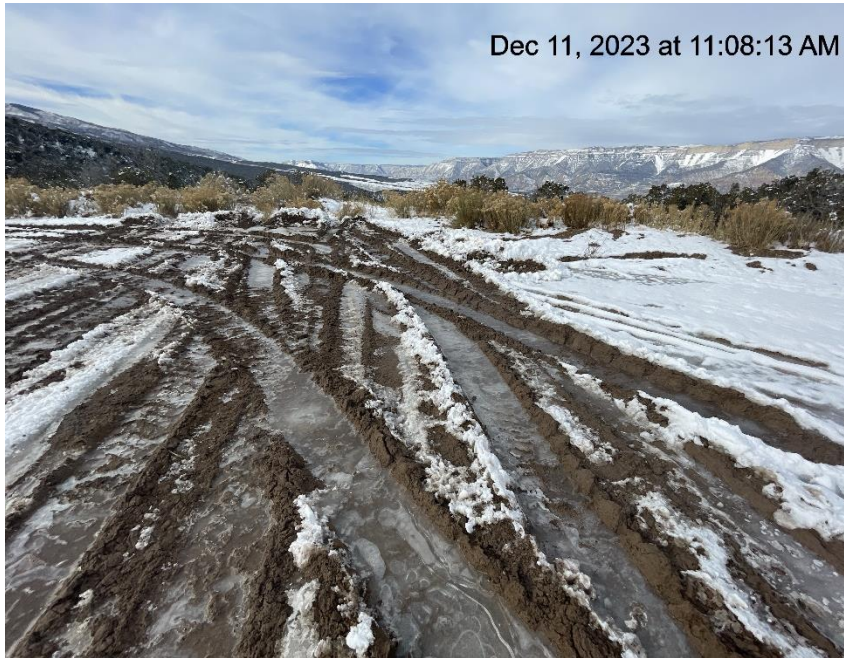
Photo # 9193 Lack of stabilization/compaction/insufficient BMP's
