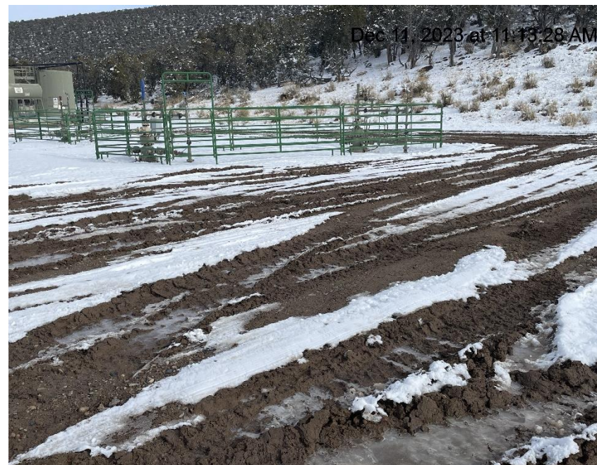
Photo # 9200 Lack of stabilization/compaction/insufficient BMP's
