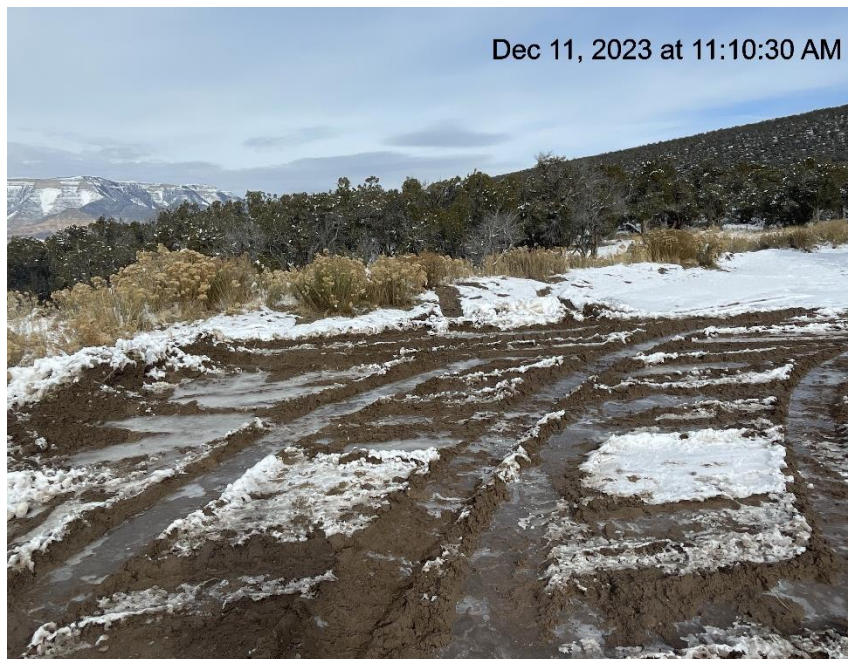
Photo # 9199 Lack of stabilization/compaction/insufficient BMP's
