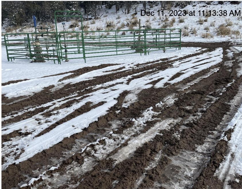
Photo # 9201 Lack of stabilization/compaction/insufficient BMP's
