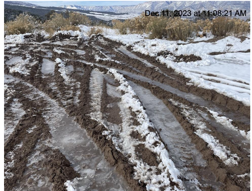
Photo # 9194 Lack of stabilization/compaction/insufficient BMP's
