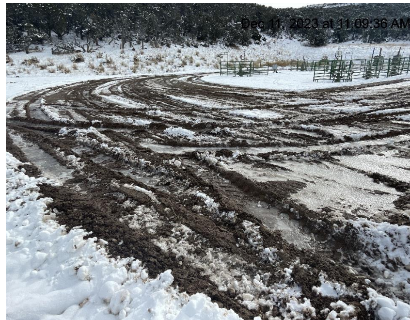
Photo # 9198 Lack of stabilization/compaction/insufficient BMP's
