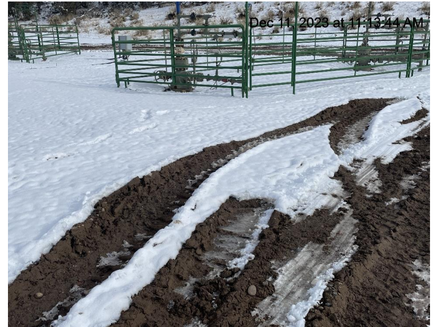
Photo # 9202 Lack of stabilization/compaction/insufficient BMP's
