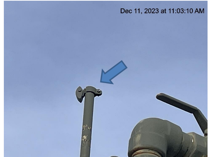
Photo # 9192 PRV vent line lacks cap
