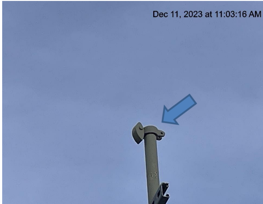
Photo # 9191 PRV vent line lacks cap
