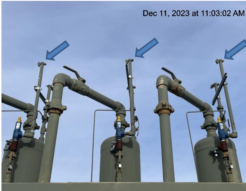
Photo # 9189 PRV vent lines lack caps
