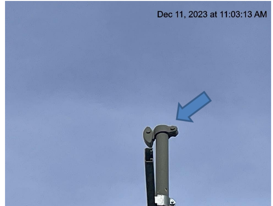
Photo # 9190 PRV vent line lacks cap
