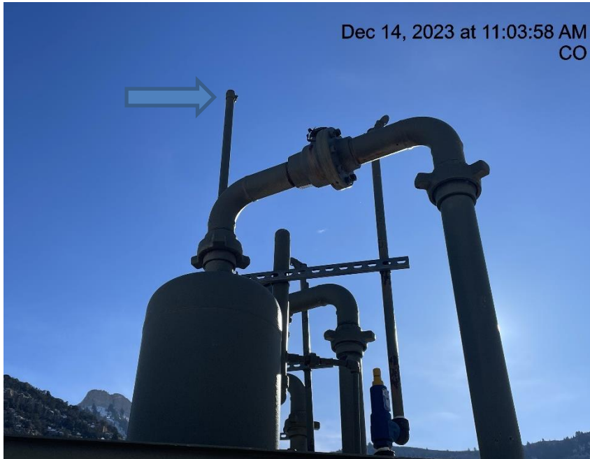
Photo # 9753 Rupture disc vent line lacks cap
