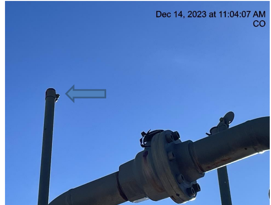
Photo # 9754 Rupture disc vent line lacks cap
