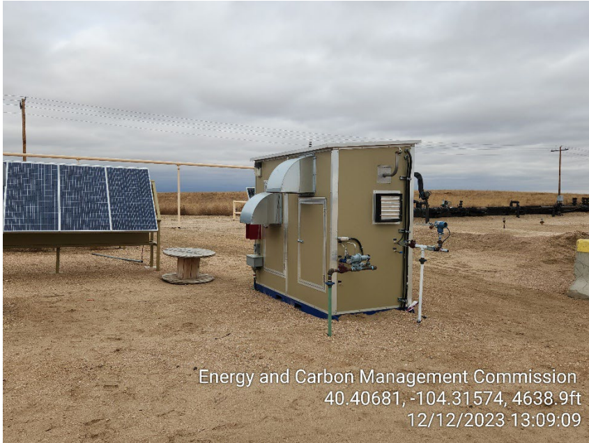
Photo 15 – Instrumental Air Unit
