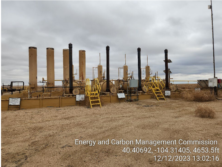
Photo 1 – Separators and ECDs
