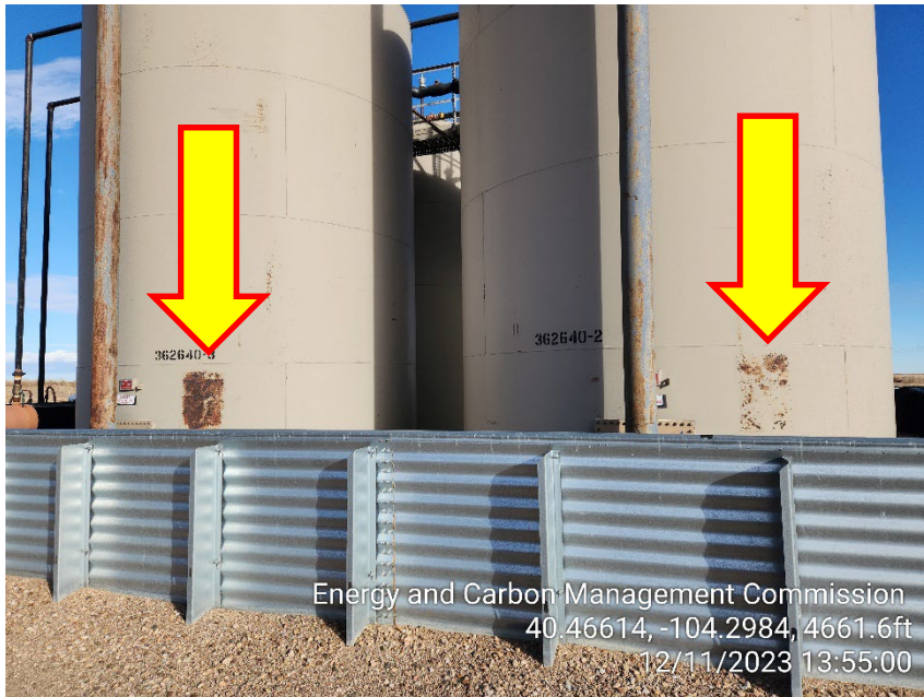
Photo 3 – Tank Labels missing
