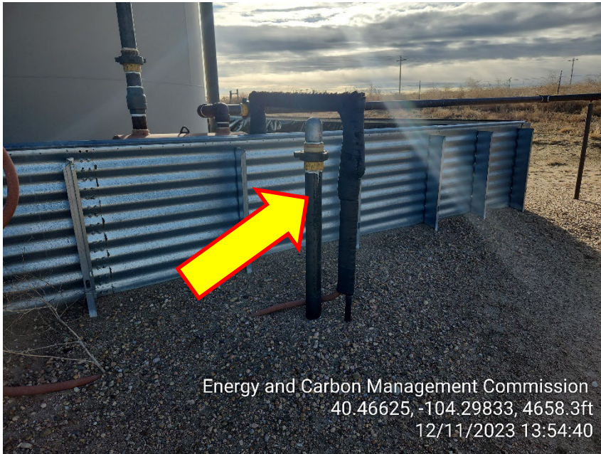
Photo 5 – 3" Riser at Tank not OOSLAT
