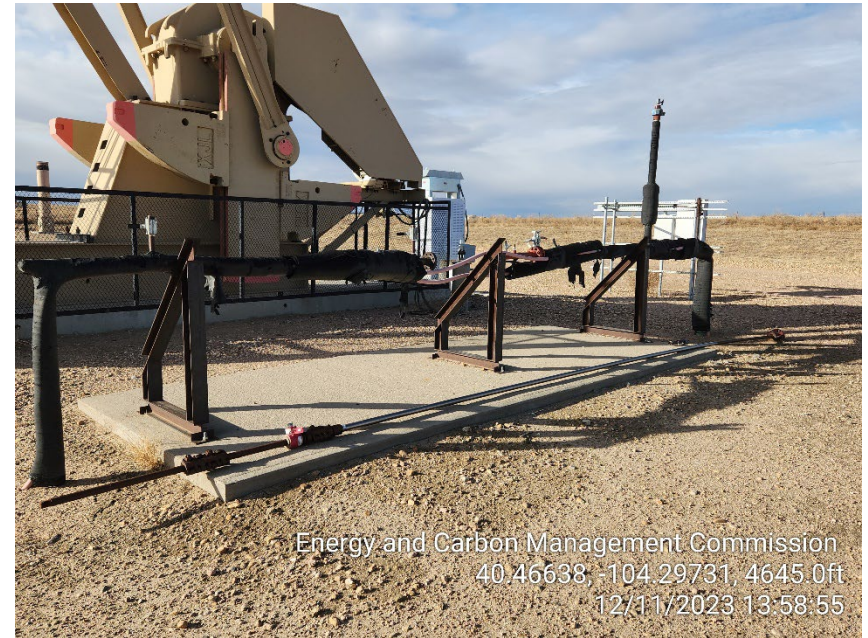
Photo 12 – Pipe Rack at Pumping Unit
