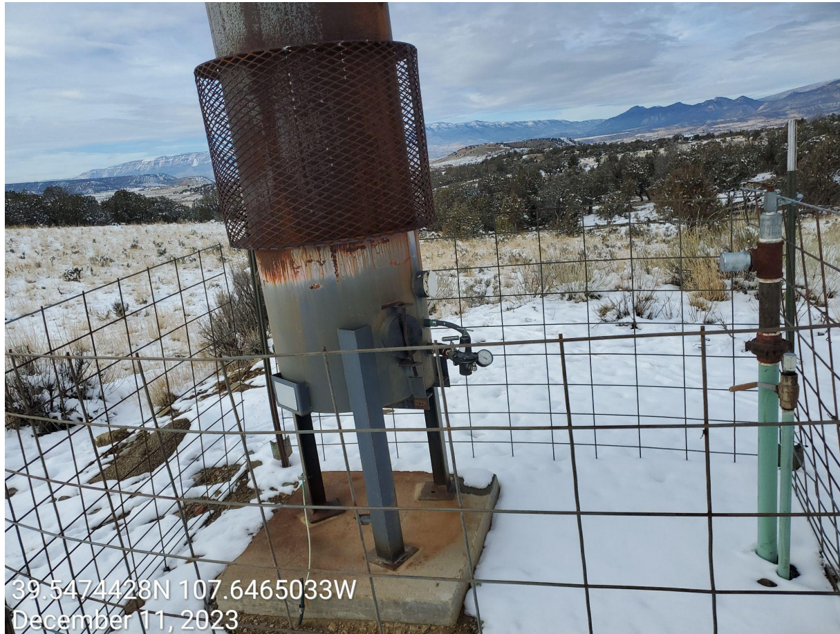
Photo 4: Photo taken from the west end of the battery site. Photo shows ECD on the Location is disconnected and not in use. Unused equipment requires removal.
