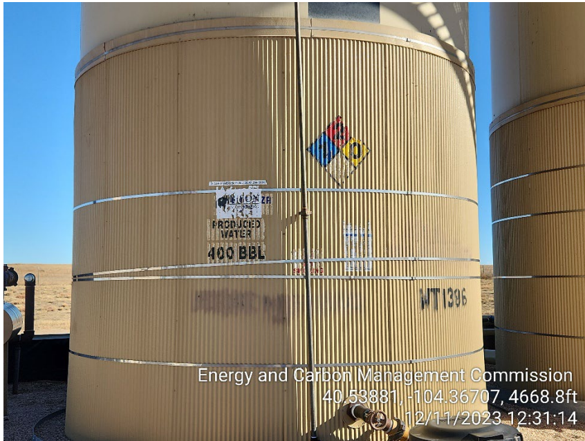
Photo 7 – Water Tank Labels – Content, Capacity, NFPA
