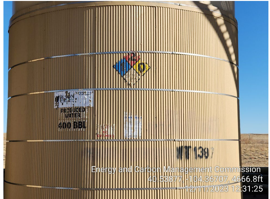
Photo 8 – Water Tank Labels – Content, Capacity, NFPA
