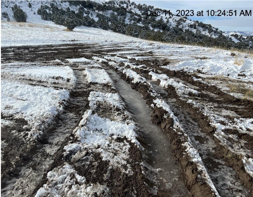
Photo # 9055 Lack of stabilization/compaction/insufficient BMP's
