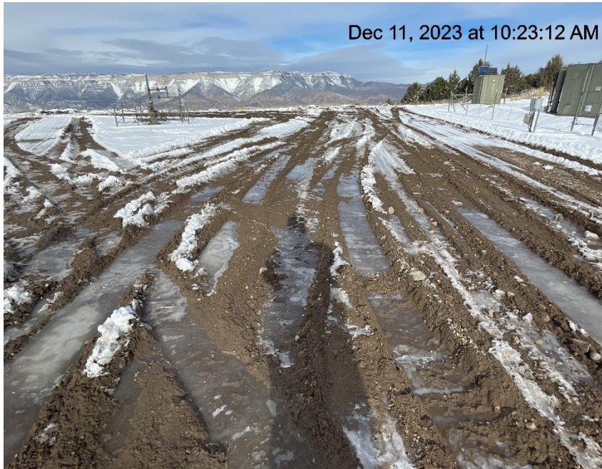
Photo # 9053 Lack of stabilization/compaction/insufficient BMP's
