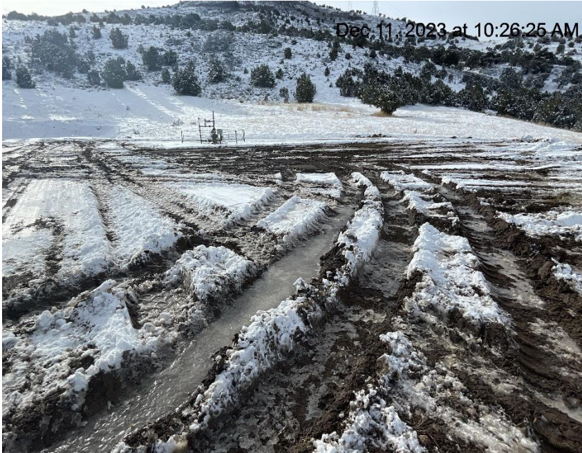
Photo # 9063 Lack of stabilization/compaction/insufficient BMP's
