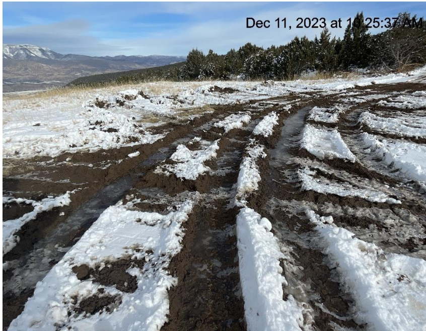
Photo # 9061 Lack of stabilization/compaction/insufficient BMP's
