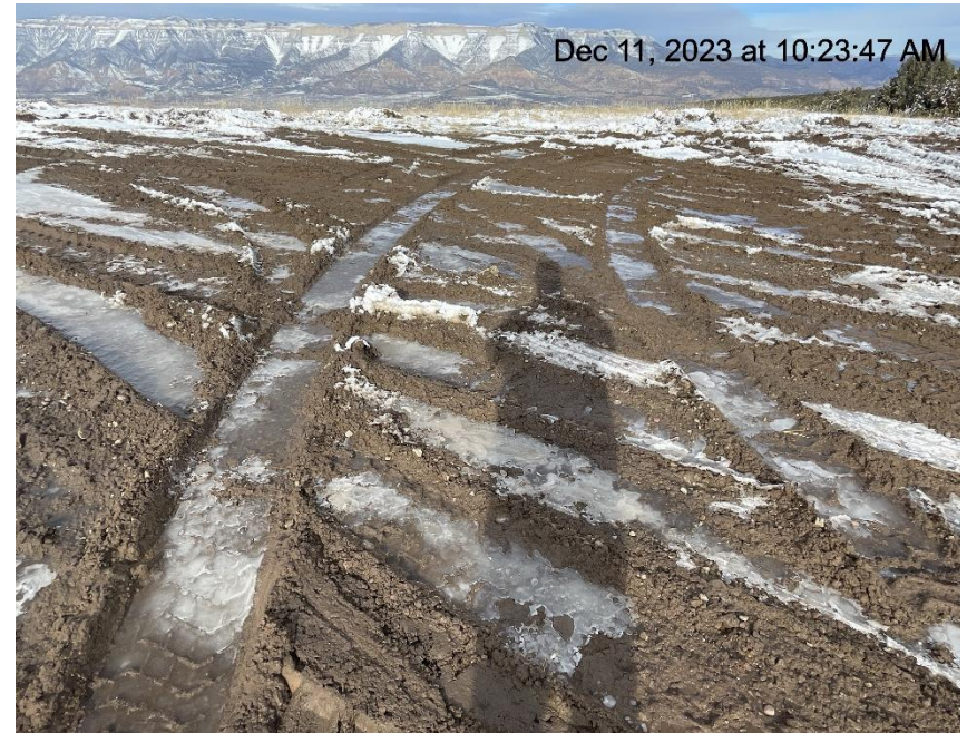
Photo # 9054 Lack of stabilization/compaction/insufficient BMP's
