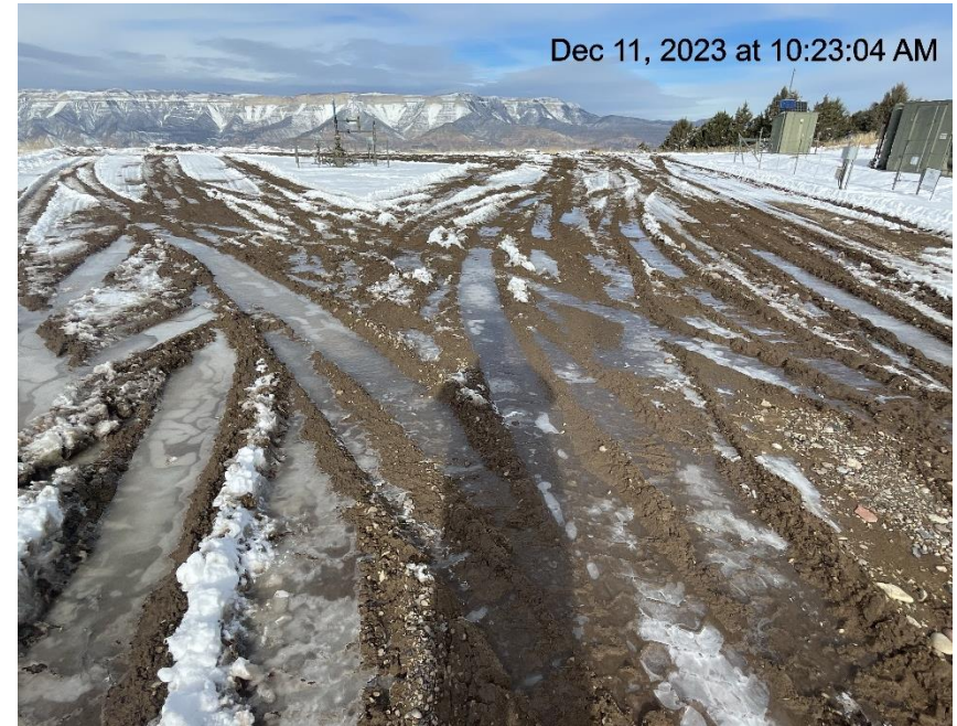
Photo # 9052 Lack of stabilization/compaction/insufficient BMP's
