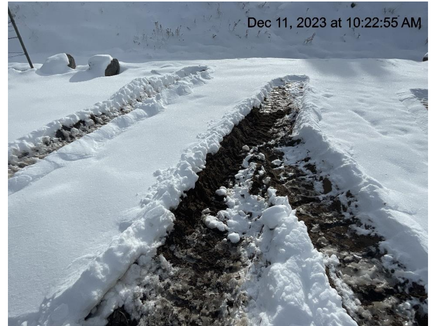
Photo # 9050 Lack of stabilization/compaction/insufficient BMP's
