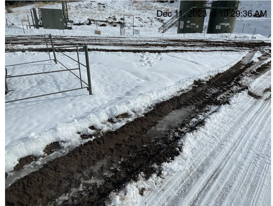
Photo #9064 Lack of stabilization/compaction/insufficient BMP's
