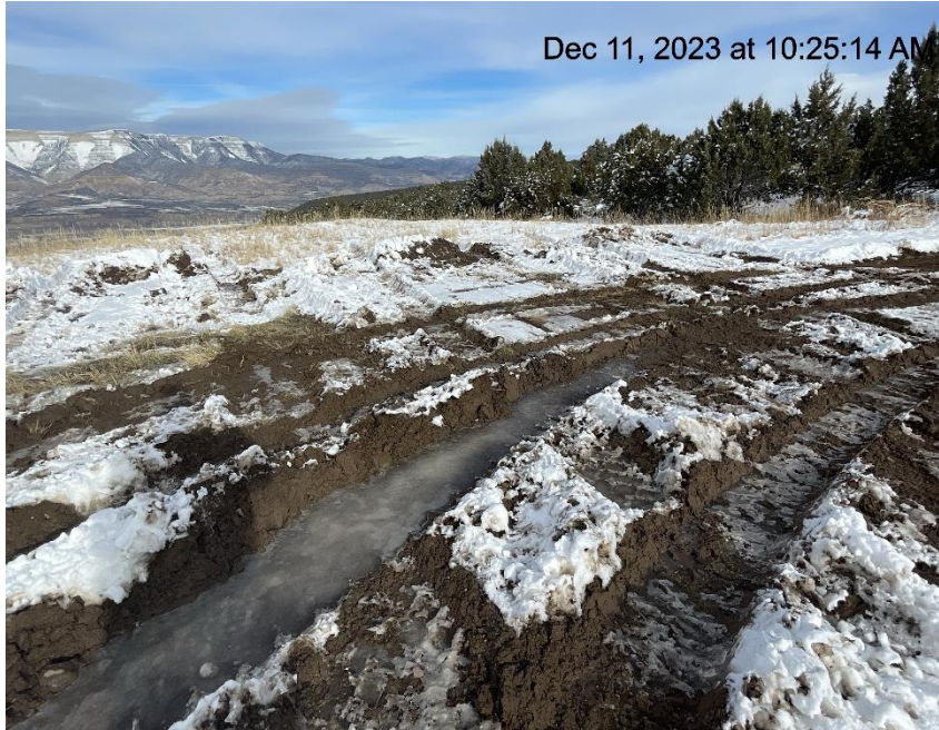
Photo # 9059 Lack of stabilization/compaction/insufficient BMP's
