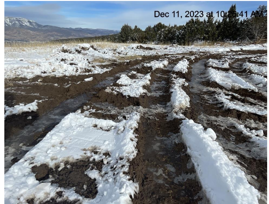
Photo # 9062 Lack of stabilization/compaction/insufficient BMP's
