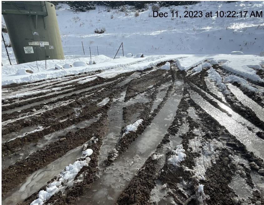
Photo # 9049 Lack of stabilization/compaction/insufficient BMP's
