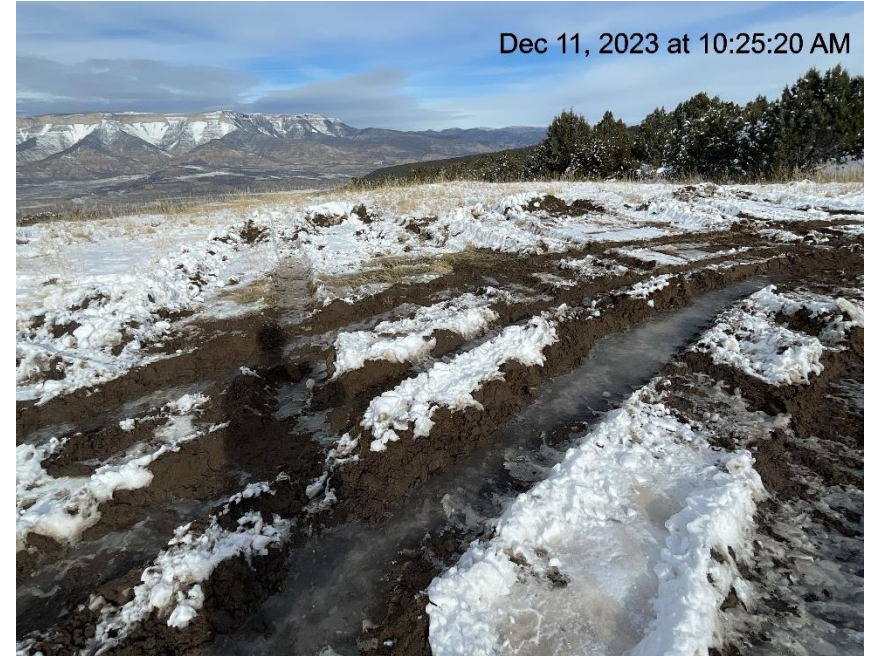
Photo # 9060 Lack of stabilization/compaction/insufficient BMP's
