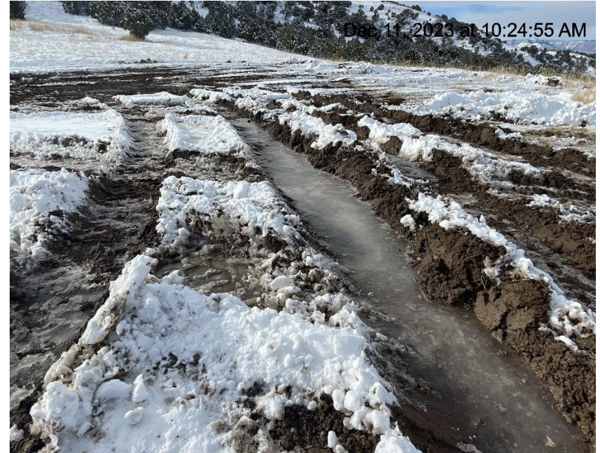
Photo # 9056 Lack of stabilization/compaction/insufficient BMP's
