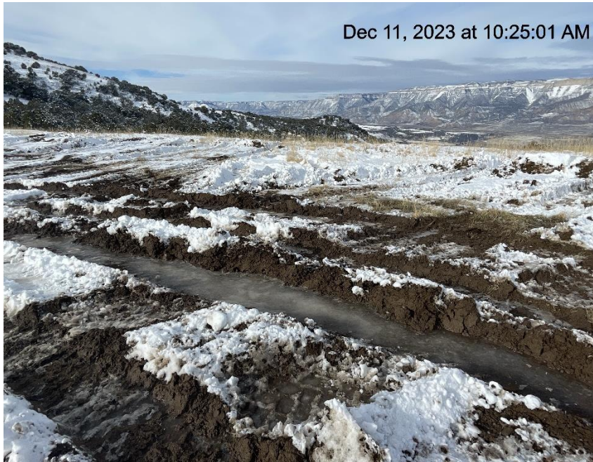
Photo # 9057 Lack of stabilization/compaction/insufficient BMP's
