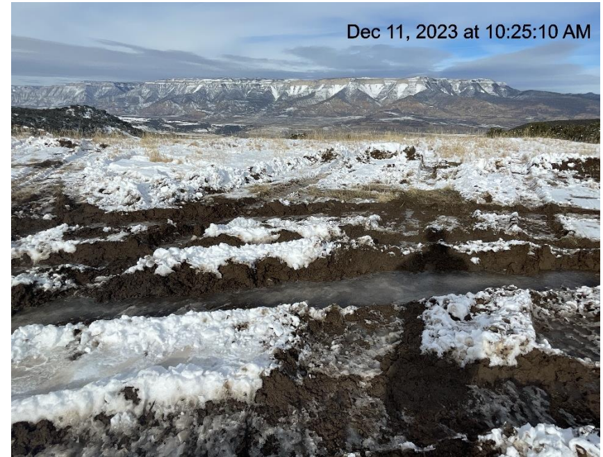
Photo # 9058 Lack of stabilization/compaction/insufficient BMP's
