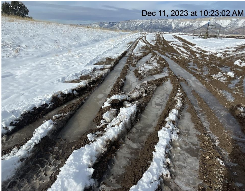
Photo # 9051 Lack of stabilization/compaction/insufficient BMP's
