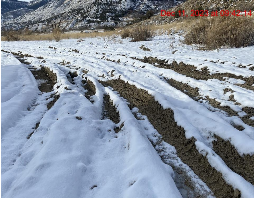
Lack of Stabilization – Photo #08040
