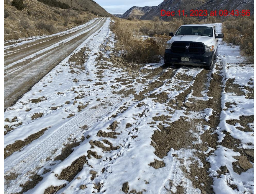
Insufficient Vehicle Tracking BMPs at Location Entrance/Exit – Photo #08041
