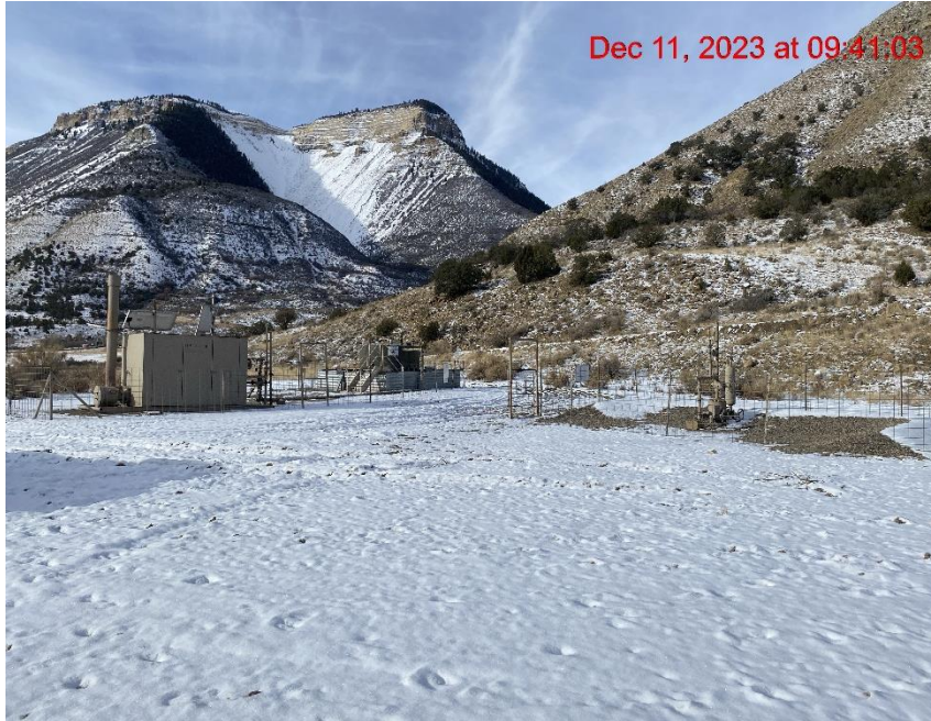
NE End of Location – Photo #08035
