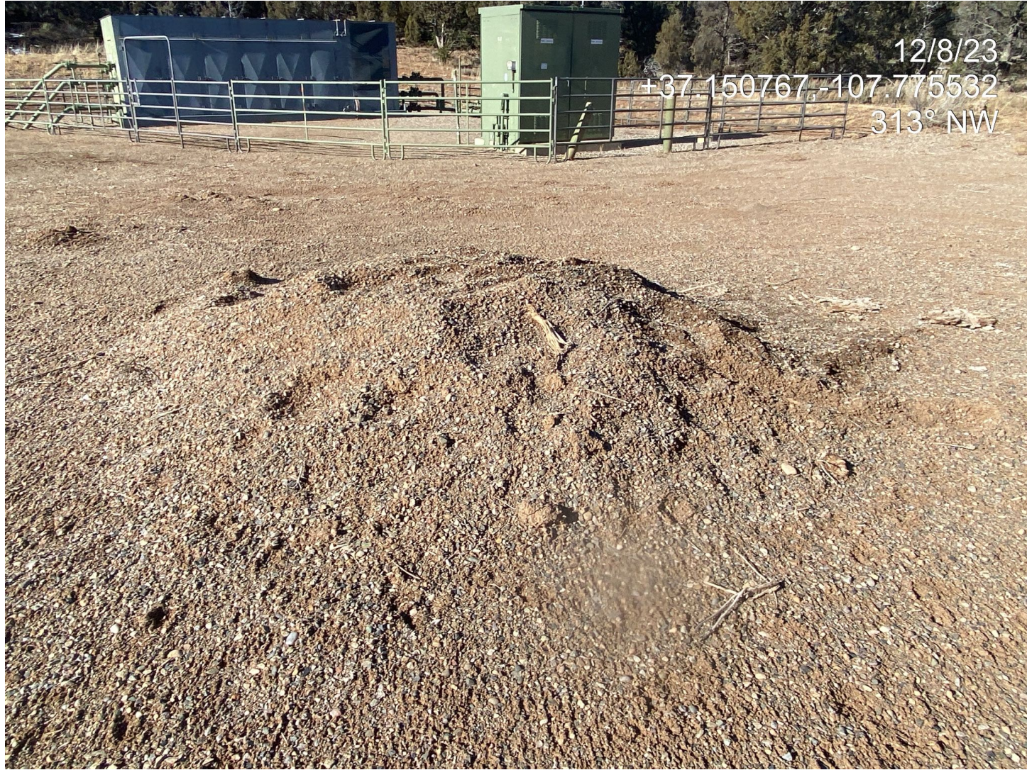
Photo 4. Pile of gravel observed on location, this is considered debris and needs to be removed.
