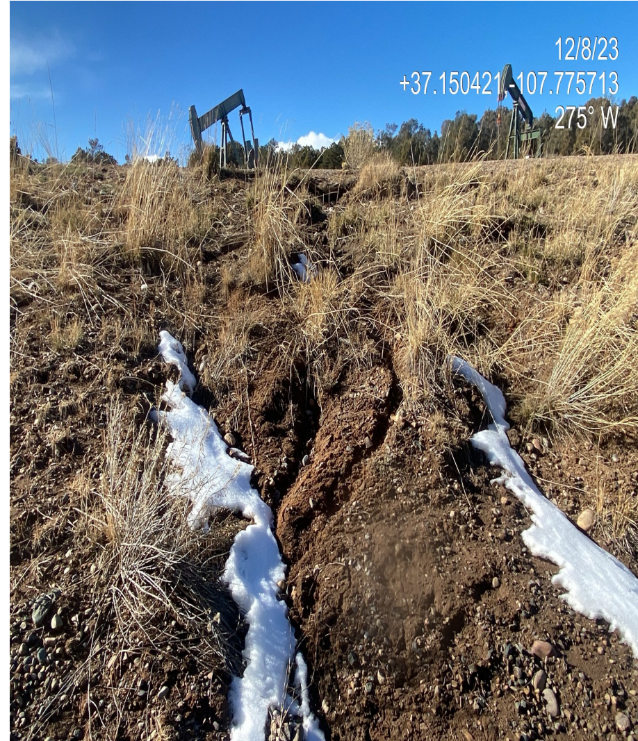
Photo 3. View of failing storm water BMPs and additional rill erosion forming in the eastern interim reclamation area.
